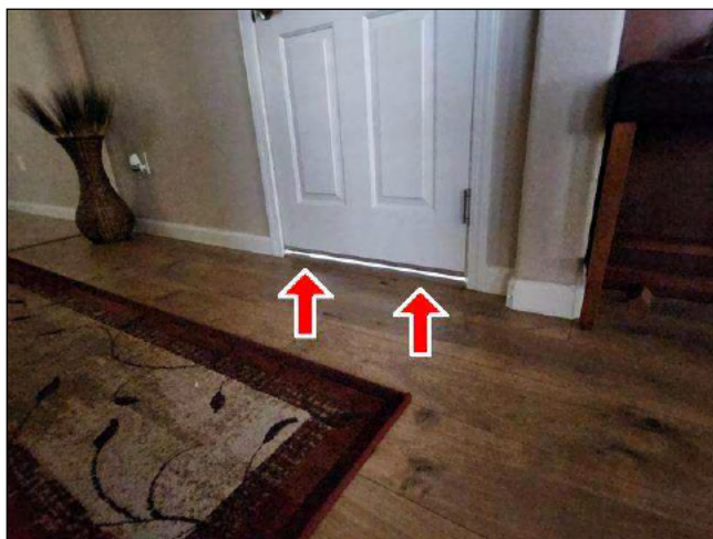
8.7 Item 1(Picture) lower seal at garage occupant door
