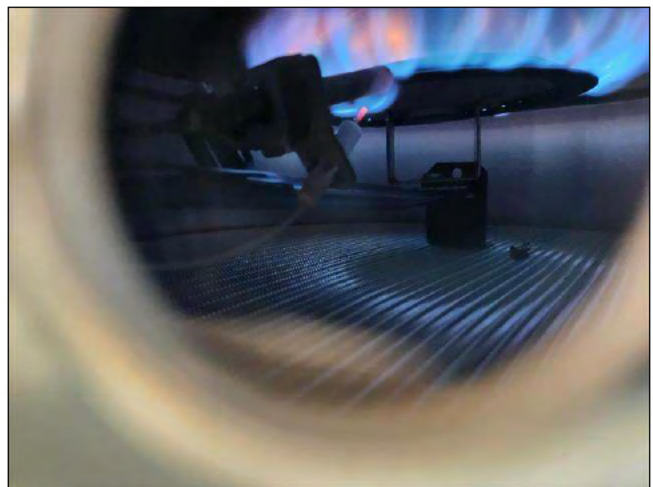
5.4 Item 2(Picture) water heater burner compartment
