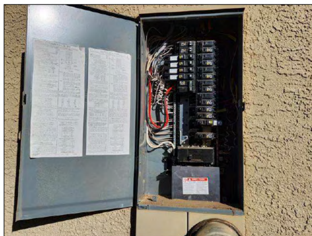
4.1 Item 2(Picture) main panel conductors
