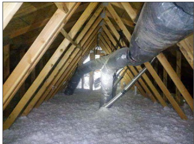
9.0 Item 2(Picture) view of attic insulation
