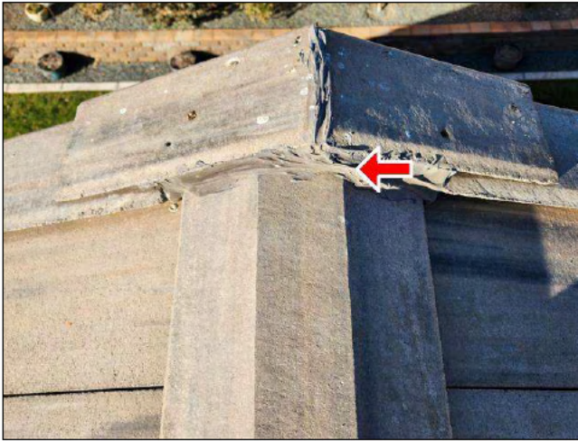
2.1 Item 3(Picture) intersecting ridges sealed well
