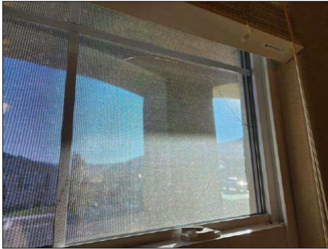
1.4 Item 1(Picture) cracked window at office
