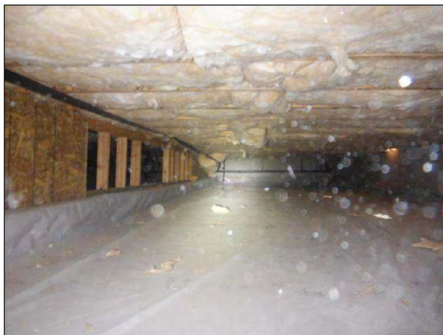
9.1 Item 1(Picture) view of subfloor insulation
