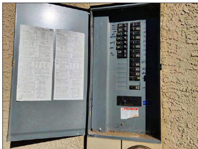
4.1 Item 1(Picture) main electrical panel
