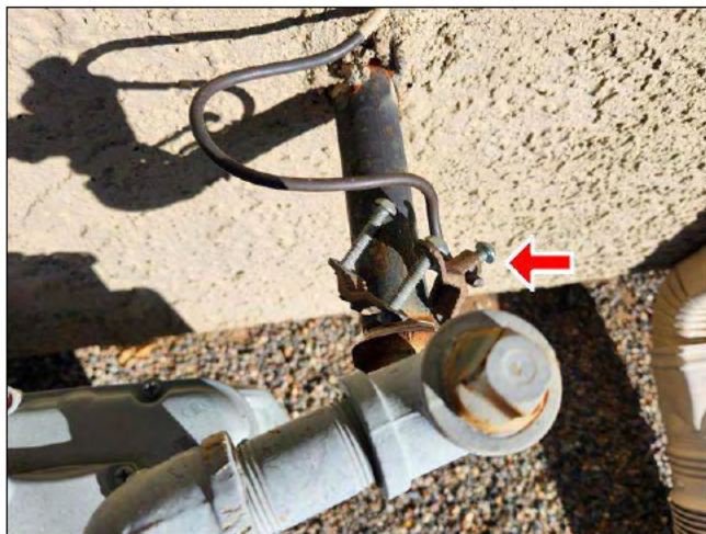
4.3 Item 1(Picture) UFER bond wire/clamp
