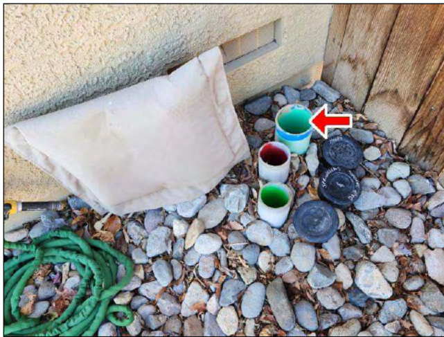
5.0 Item 1(Picture) main water shut-off valve location
