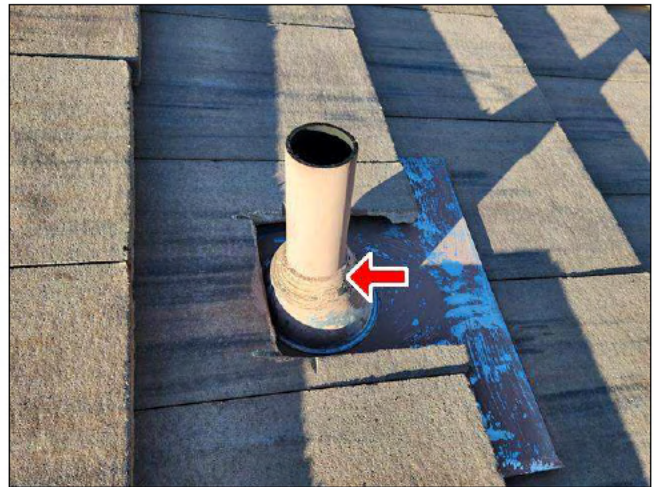
2.3 Item 2(Picture) plumbing vent pipes sealed well
