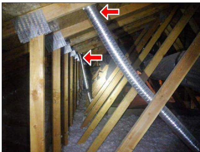
9.4 Item 1(Picture) vented properly to exterior
