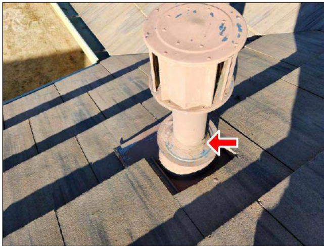
2.3 Item 1(Picture) flue pipes sealed well
