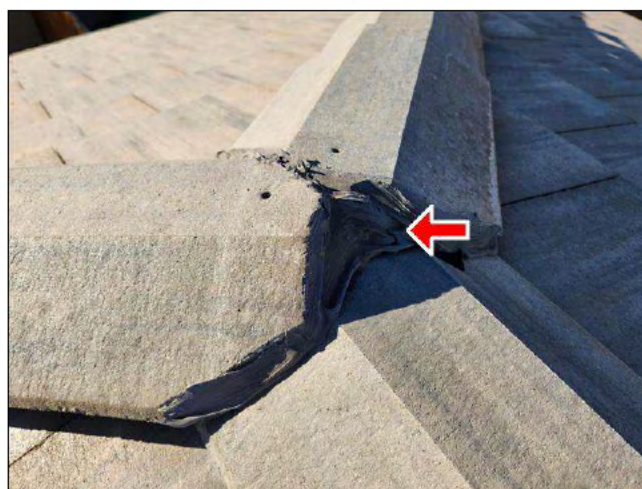
2.1 Item 2(Picture) intersecting ridges sealed well
