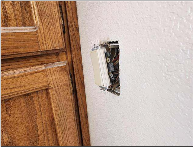
4.5 Item 1(Picture) loose electrical switch at kitchen
