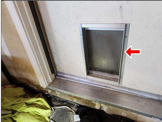
8.8 Item 1(Picture) compromised fire-separation door
