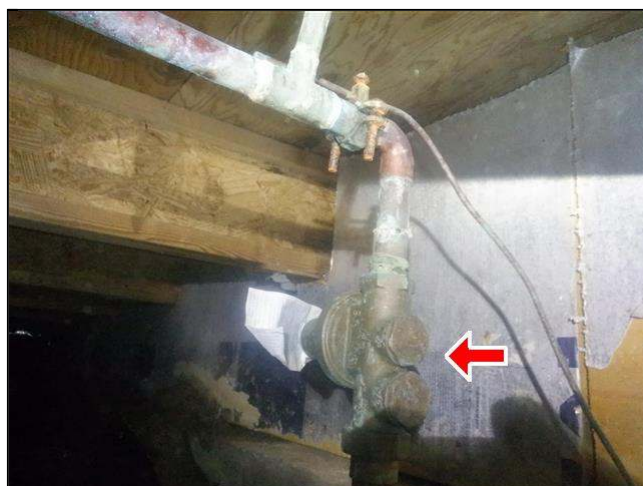
5.2 Item 6(Picture) pressure regulator in crawlspace
