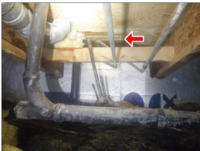
5.2 Item 3(Picture) wet subfloor under laundry room
