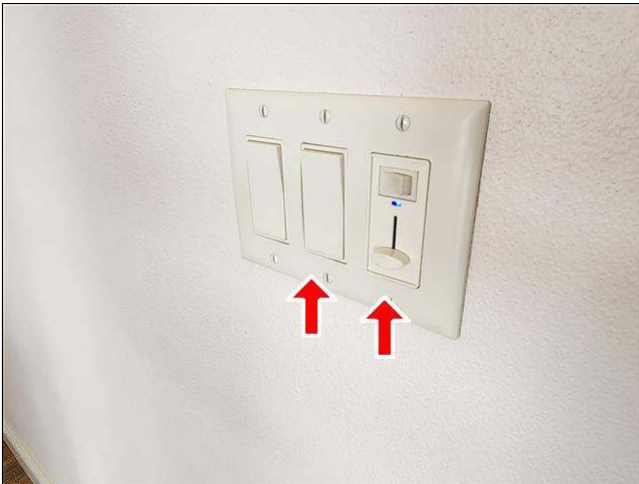
4.5 Item 2(Picture) both switches operate ceiling light
