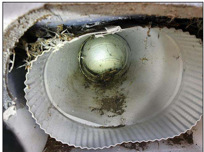
9.4 Item 2(Picture) open for pest access
