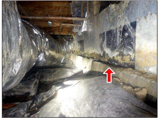
3.2 Item 4(Picture) moisture intrusion at south foundation
