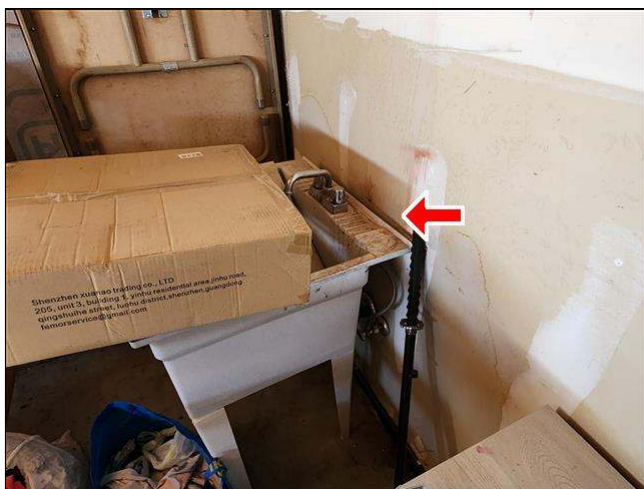
5.5 Item 1(Picture) utility sink not secured
