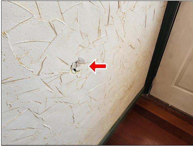
7.2 Item 1(Picture) drywall repair needed at main entry
