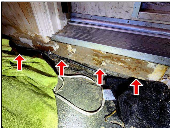
5.2 Item 1(Picture) moisture dripping at garage occupant door area
