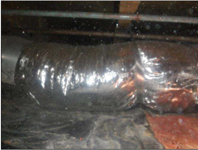
10.3 Item 1(Picture) wet duct on crawlspace ground
