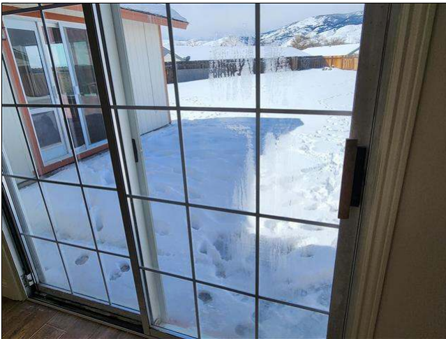
1.4 Item 1(Picture) condensation at master bedroom slider door
