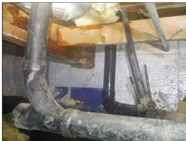
5.2 Item 4(Picture) wet subfloor under laundry room
