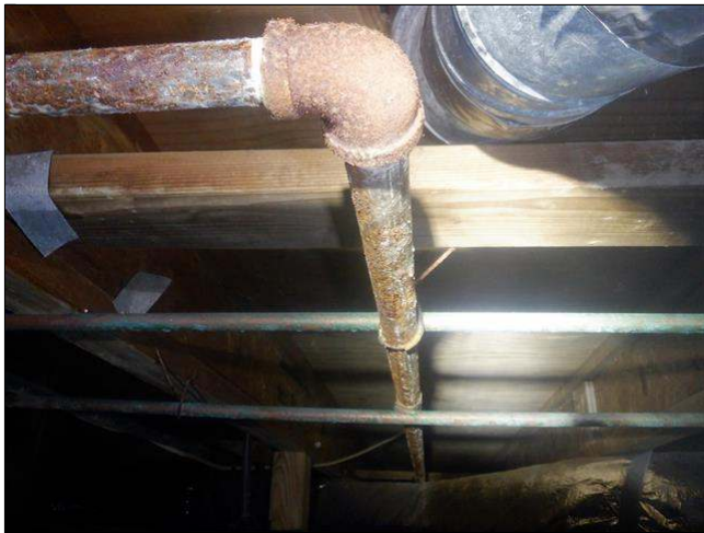
9.3 Item 1(Picture) rust on gas supply pipes
