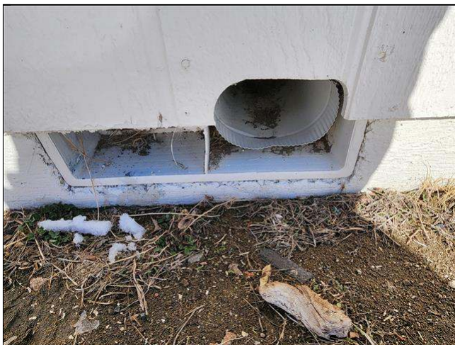
9.4 Item 1(Picture) open vent for kitchen range
