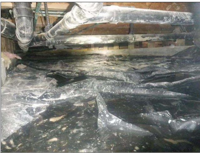
3.2 Item 5(Picture) pooled moisture in crawlspace
