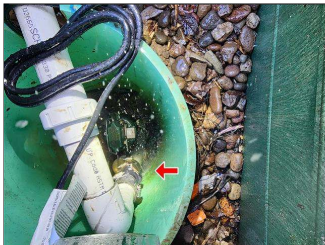
5.12 Item 2(Picture) pumping water back into the pump well
