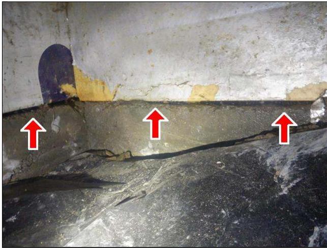
3.2 Item 1(Picture) moisture intrusion at right rear corner
