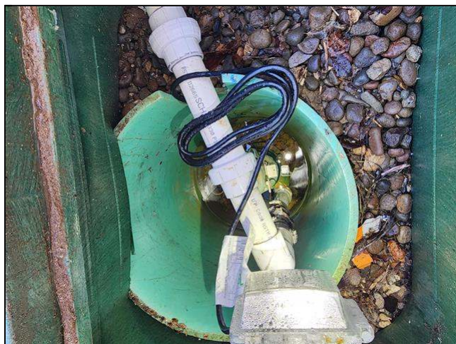
5.12 Item 1(Picture) north exterior sump pump
