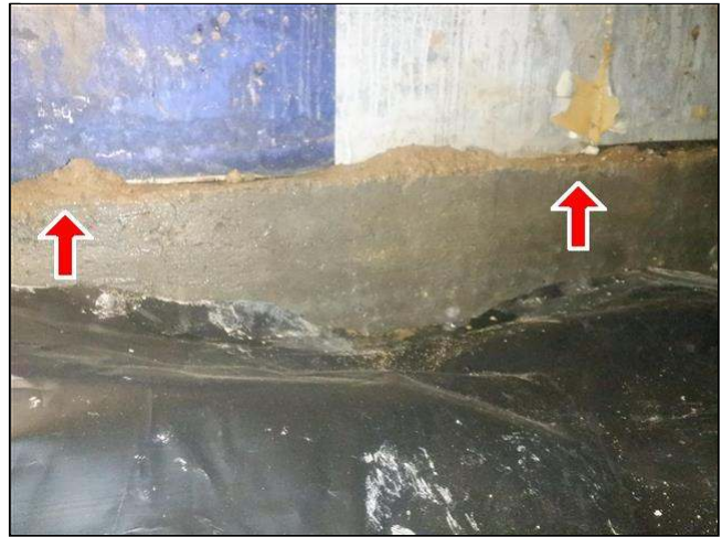
3.2 Item 2(Picture) moisture intrusion at right rear corner
