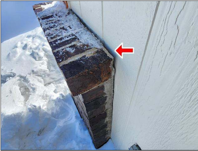
1.1 Item 3(Picture) bricks pulled away at right front corner
