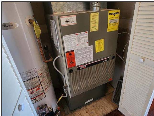
10.0 Item 1(Picture) forced air furnace
