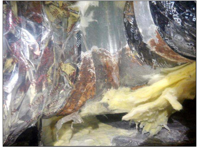
10.3 Item 2(Picture) rust on heat duct connector sleeve
