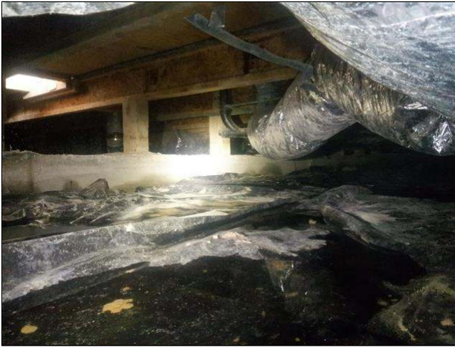
3.2 Item 3(Picture) pooled moisture in crawlspace
