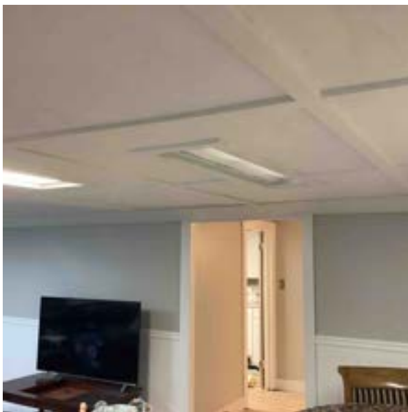
8.9.4 Replace missing/damaged light globe covers to prevent electrical hazards. (Basement Living Room)
