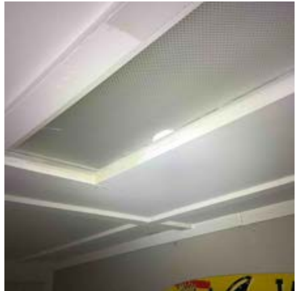
8.9.4 Replace missing/damaged light globe covers to prevent electrical hazards. (Basement Living Room)
