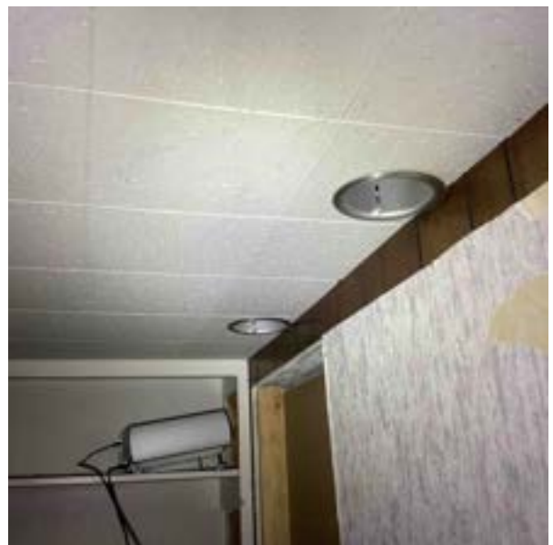
8.9.4 Replace missing/damaged light globe covers to prevent electrical hazards. (Basement Living Room)
