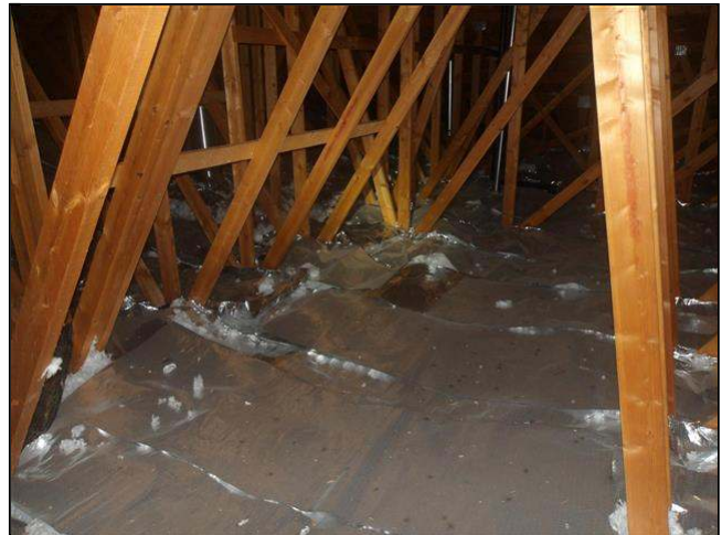
9.0 Item 2(Picture) view of attic insulation
