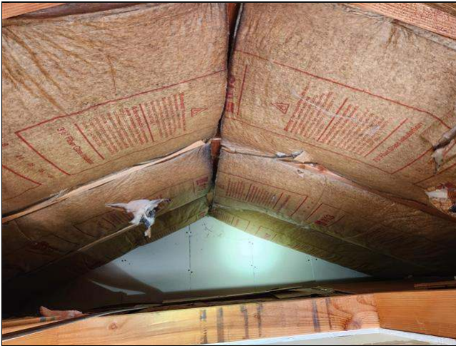
1.9 Item 3(Picture) view of roof structure and attic area
