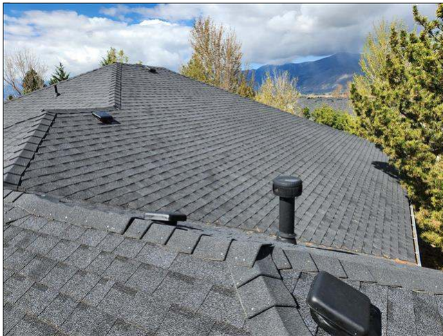
2.0 Item 1(Picture) view of roof
