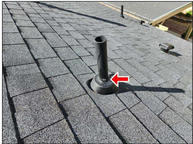
2.3 Item 2(Picture) Plumbing and furnace vent pipes are sealed well
