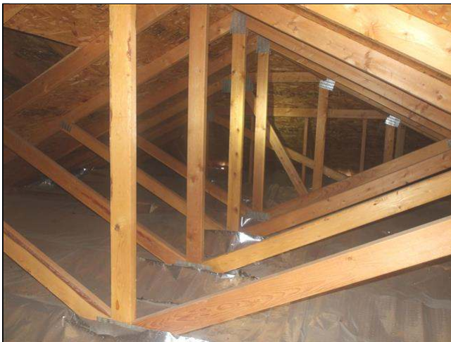
8.11 Item 1(Picture) view of garage roof structure
