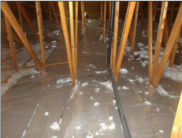
9.0 Item 1(Picture) view of attic insulation
