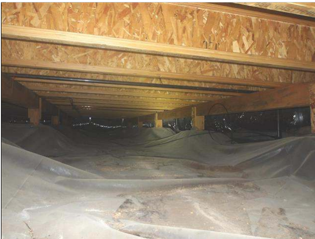
3.0 Item 7(Picture) view of crawlspace
