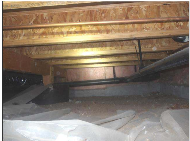
3.0 Item 8(Picture) view of crawlspace
