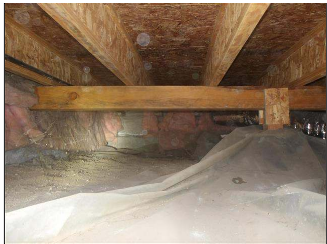
3.0 Item 2(Picture) view of crawlspace
