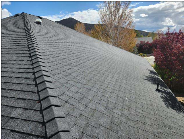
2.0 Item 3(Picture) view of roof
