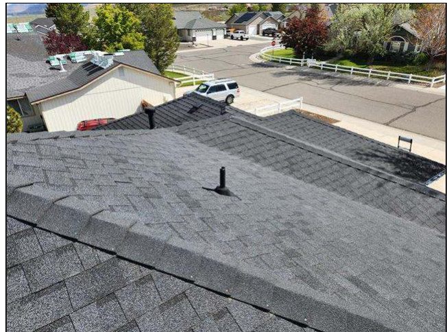
2.0 Item 4(Picture) view of roof
