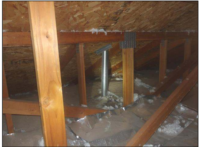
3.8 Item 6(Picture) view of attic
