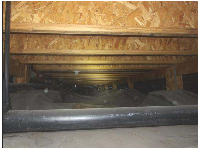
3.0 Item 6(Picture) view of crawlspace
