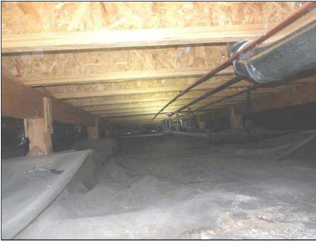
3.0 Item 3(Picture) view of crawlspace
