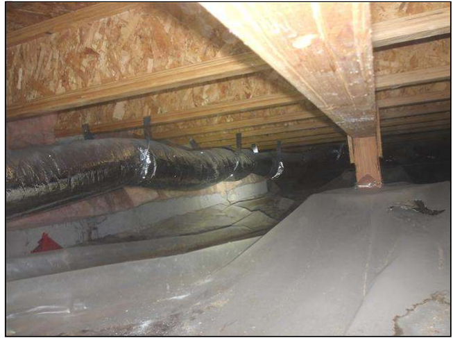
3.0 Item 4(Picture) view of crawlspace
