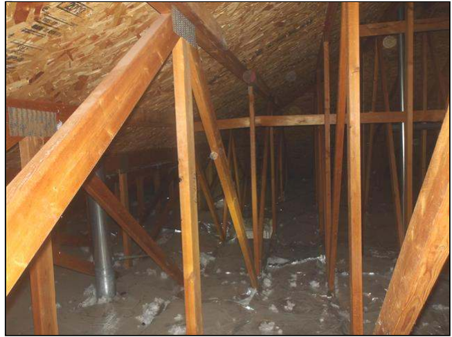
3.8 Item 4(Picture) view of attic
