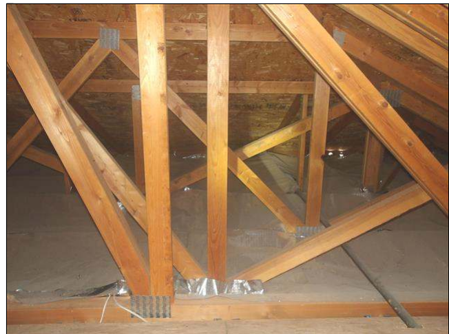
8.11 Item 2(Picture) view of garage roof structure
