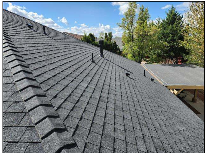
2.0 Item 2(Picture) view of roof
