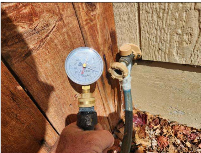
5.2 Item 1(Picture) water pressure at front hose bib
