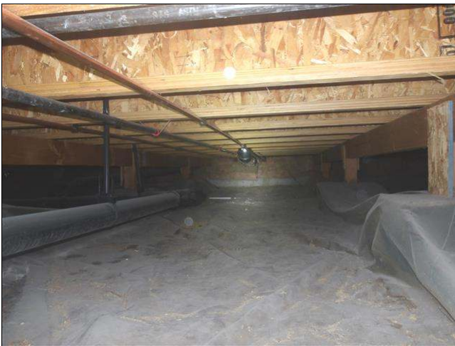
3.0 Item 1(Picture) view of crawlspace
