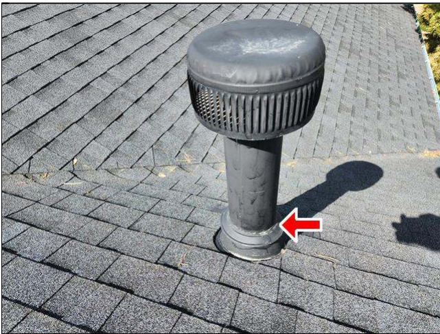
2.3 Item 1(Picture) Plumbing and furnace vent pipes are sealed well
