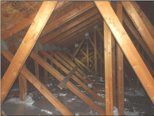
3.8 Item 5(Picture) view of attic
