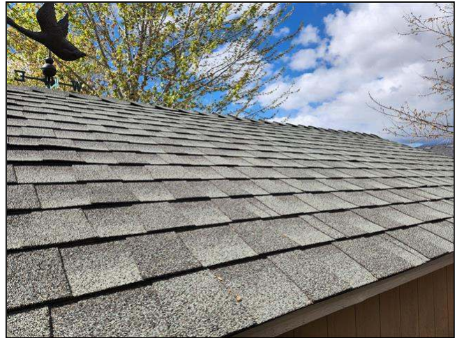
1.9 Item 4(Picture) view of roof covering
