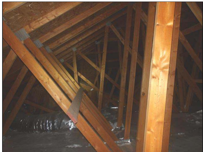
3.8 Item 2(Picture) view of attic
