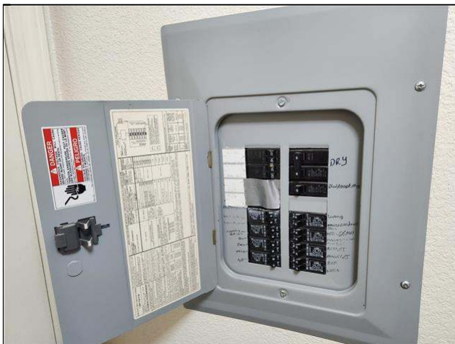
4.1 Item 1(Picture) laundry room panel
