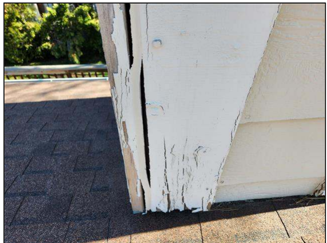
1.2 Item 4(Picture) loosened chimney trim boards
