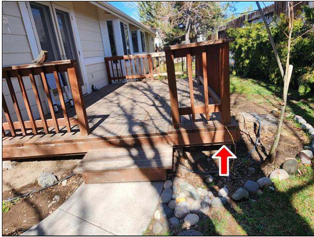
1.6 Item 1(Picture) lifted corner of rear deck
