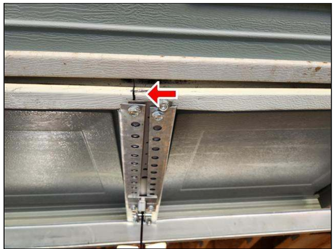
8.7 Item 2(Picture) creases at garage door panels
