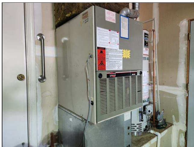
10.0 Item 1(Picture) forced air furnace
