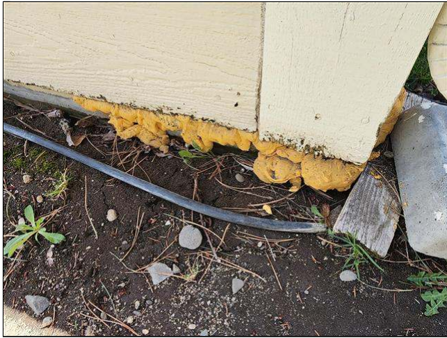
1.1 Item 6(Picture) foam/sealant at NW corner of home
