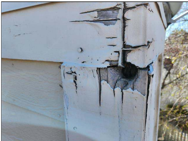
1.2 Item 3(Picture) hole through chimney trim board
