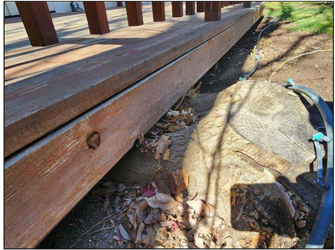
1.6 Item 2(Picture) tree root lifting deck
