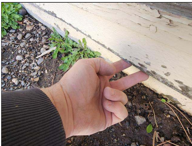
1.1 Item 5(Picture) lower edge of siding is wet
