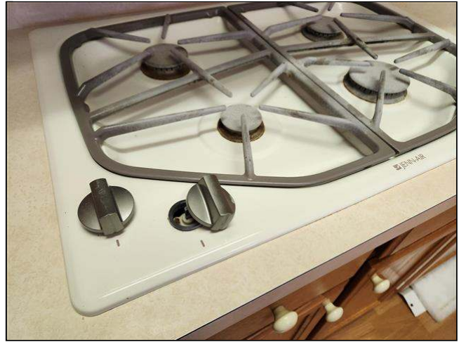
6.2 Item 2(Picture) loose/worn knobs
