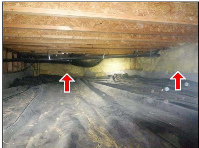
9.0 Item 2(Picture) view of crawlspace insulation
