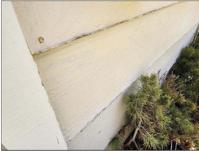
1.1 Item 1(Picture) normal wear/age on siding
