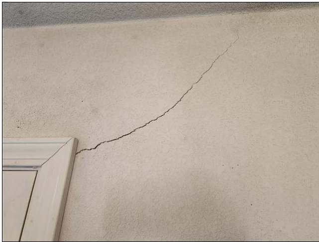
7.2 Item 1(Picture) larger settlement crack at living room
