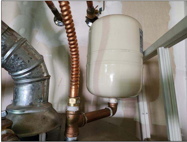
5.4 Item 3(Picture) thermal expansion tank
