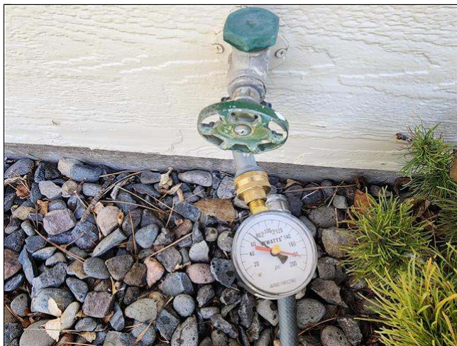
5.2 Item 1(Picture) water pressure at front hose bib
