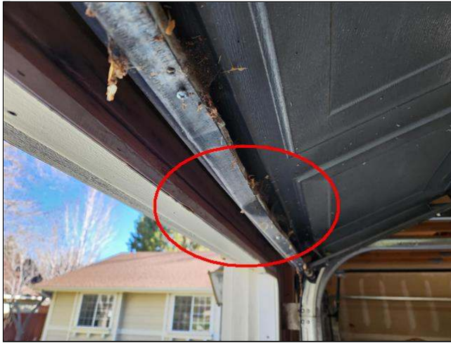
8.7 Item 3(Picture) drags framing header when opening
