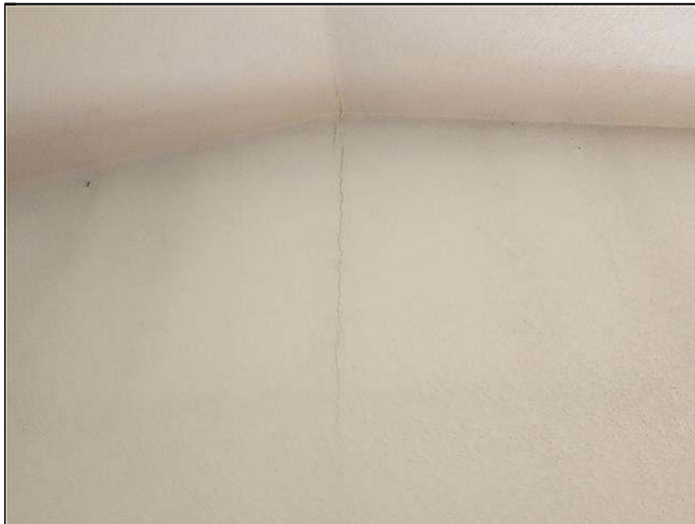
7.2 Item 3(Picture) average settlement cracks
