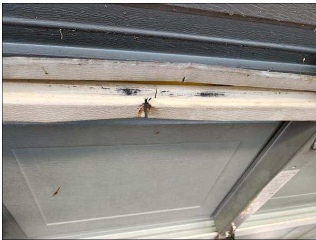
8.7 Item 1(Picture) creases at garage door panels
