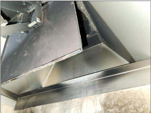
11.0 Item 2(Picture) fireplace chimney damper
