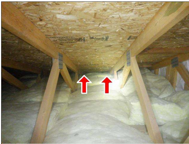
3.8 Item 1(Picture) blackening plywood at NE corner
