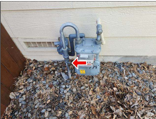
5.11 Item 1(Picture) main fuel shut-off valve
