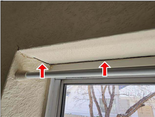
7.5 Item 1(Picture) interior window opening caulking
