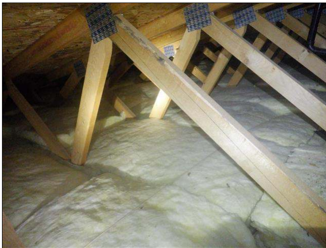
9.0 Item 1(Picture) view of attic insulation
