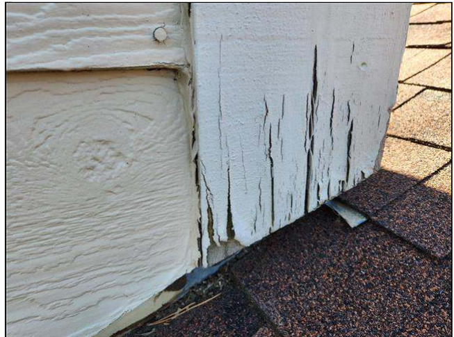
1.2 Item 2(Picture) cracked chimney trim boards
