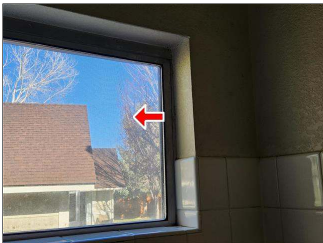
1.4 Item 3(Picture) cracked window panel
