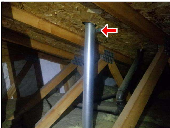
9.4 Item 1(Picture) properly vented to exterior
