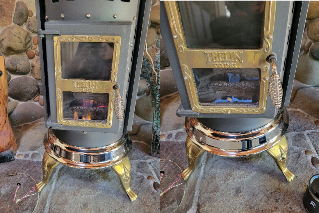
10.0 of Home Inspection Report —Seller repaired freestanding gas log fireplace to respond to normal operating controls with gas valves in the ON position. Seller replaced a bad thermopile.
