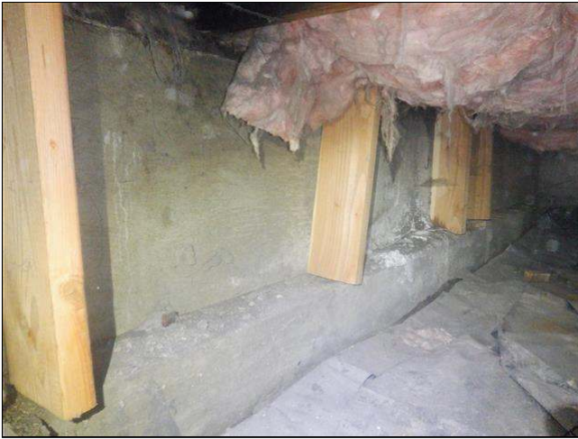
3.4 Item 1(Picture) additional support posts installed
