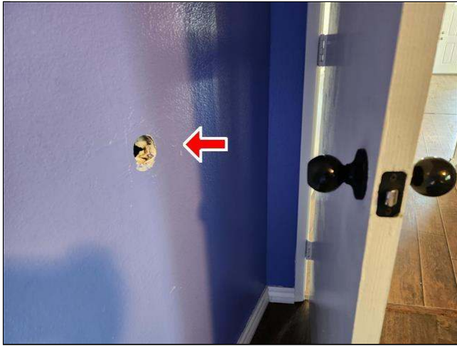
7.2 Item 1(Picture) drywall damage at NE bedroom
