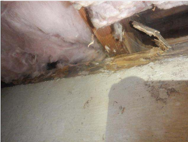
3.2 Item 7(Picture) moisture affected sole plate
