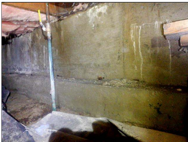
3.2 Item 1(Picture) moisture at north foundation
