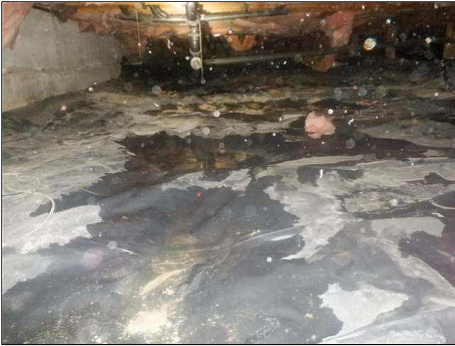
3.2 Item 3(Picture) pooled moisture at south side
