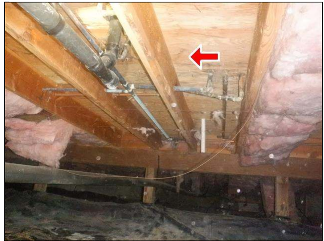
8.1 Item 2(Picture) missing insulation under bathroom
