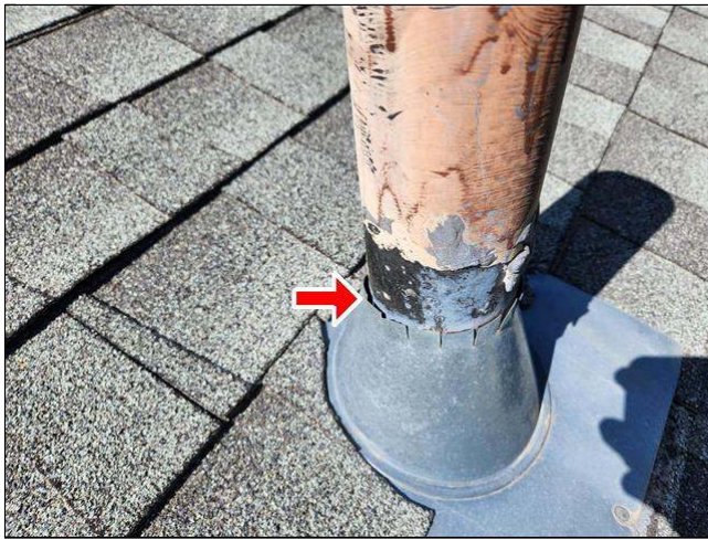
2.3 Item 1(Picture) seal main soil stack
