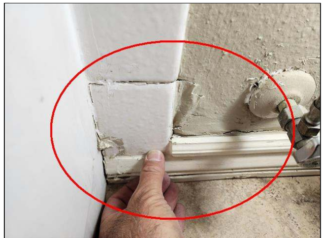
5.6 Item 3(Picture) moisture damaged drywall area
