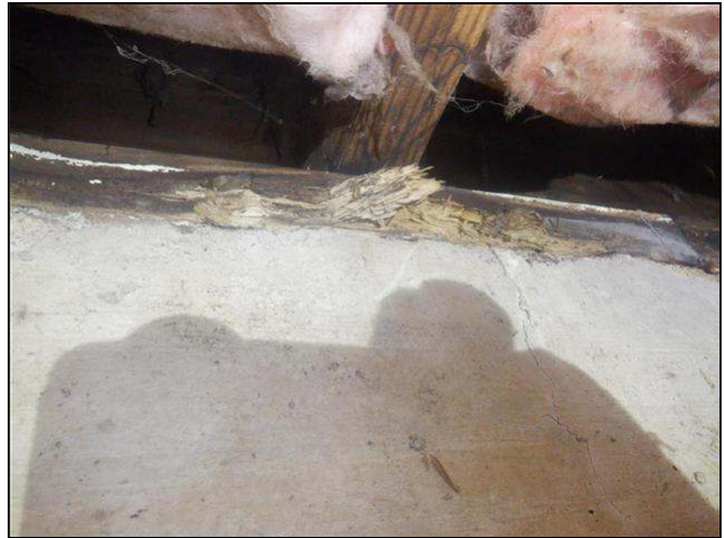
3.2 Item 6(Picture) moisture affected sole plate
