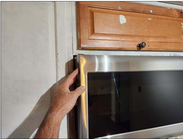
6.5 Item 1(Picture) microwave not properly supported
