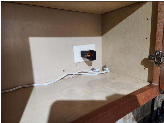
4.5 Item 1(Picture) open grounded outlets
