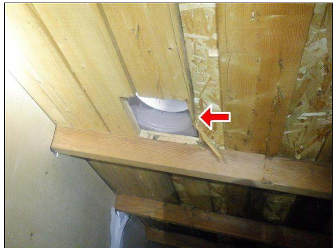
8.3 Item 2(Picture) additional roof vents installed
