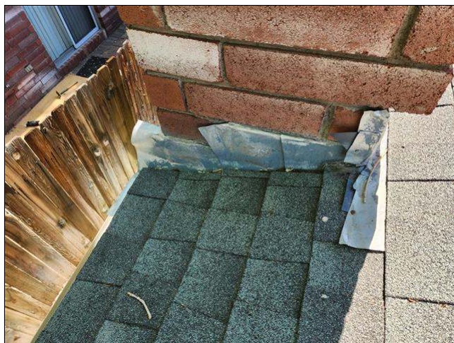
10.1 Item 2(Picture) chimney flashings
