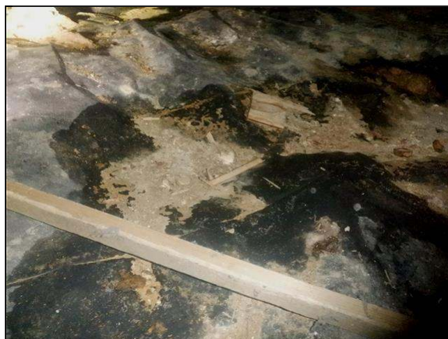
5.2 Item 2(Picture) moisture from leak
