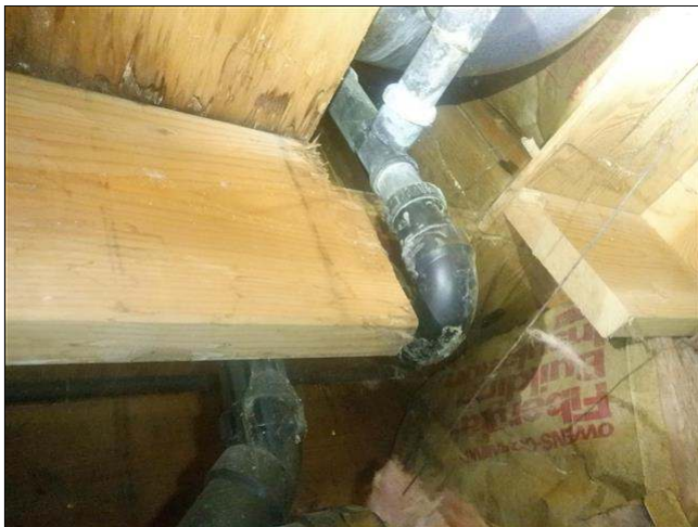
3.6 Item 2(Picture) cut joist under master bath
