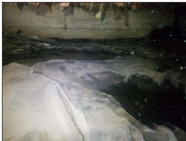
3.2 Item 2(Picture) pooled moisture at north side
