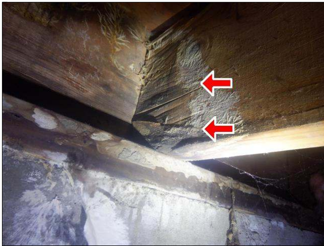
3.6 Item 4(Picture) soft joist from moisture
