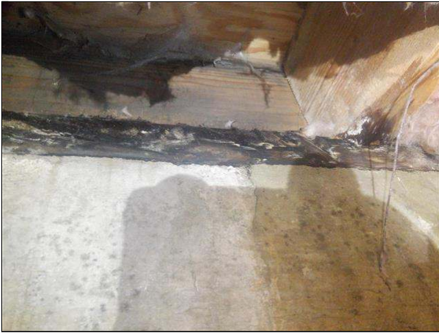
3.2 Item 9(Picture) moisture affected sole plate
