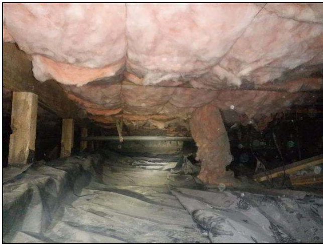
3.6 Item 1(Picture) subfloor covered with insulation
