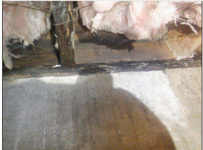
3.2 Item 8(Picture) moisture affected sole plate
