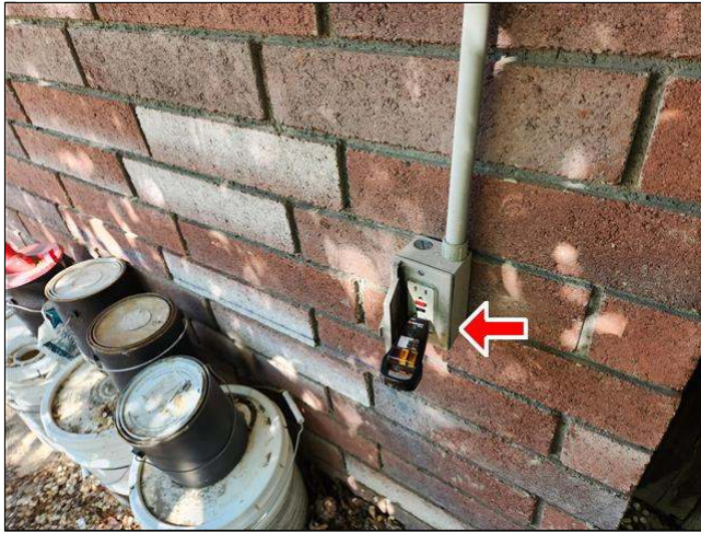
4.7 Item 1(Picture) faulty gfci at rear exterior
