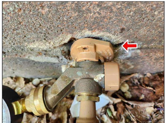
5.0 Item 2(Picture) secure and seal flange
