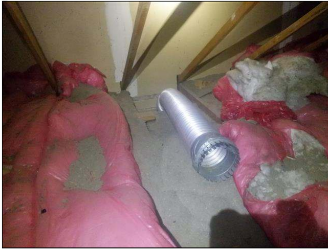
8.4 Item 1(Picture) kitchen vents into attic
