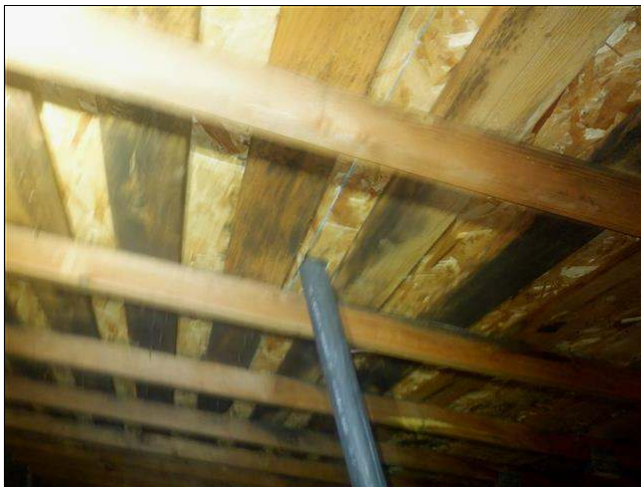
8.3 Item 1(Picture) blackening of roof boards
