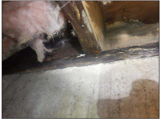
3.2 Item 10(Picture) moisture affected sole plate
