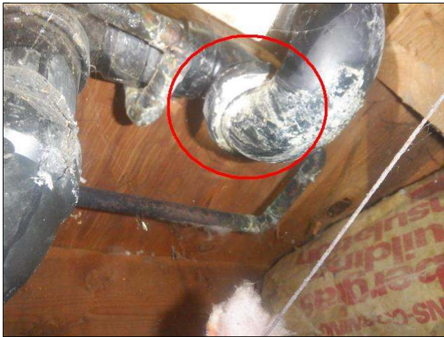
5.2 Item 3(Picture) leaking drain under master tub
