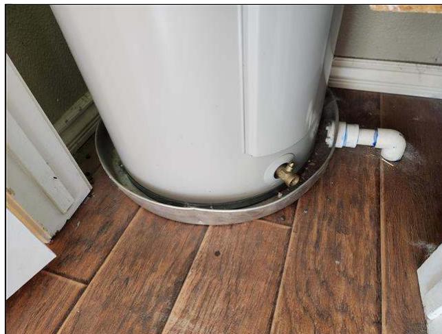
5.3 Item 2(Picture) setting in a drip pan
