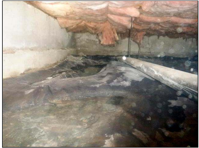
3.2 Item 4(Picture) pooled moisture at SW corner
