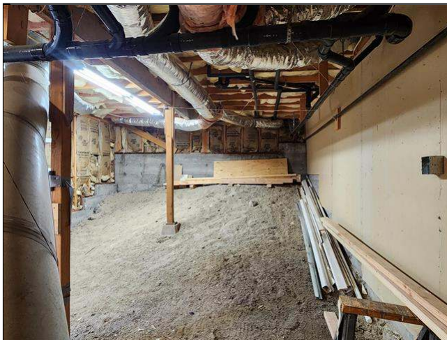
3.0 Item 1(Picture) view of crawlspace
