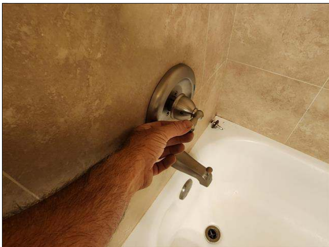
5.5 Item 1(Picture) downstairs shower control valves
