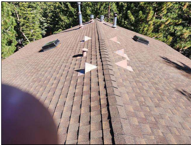
2.0 Item 1(Picture) view of roof
