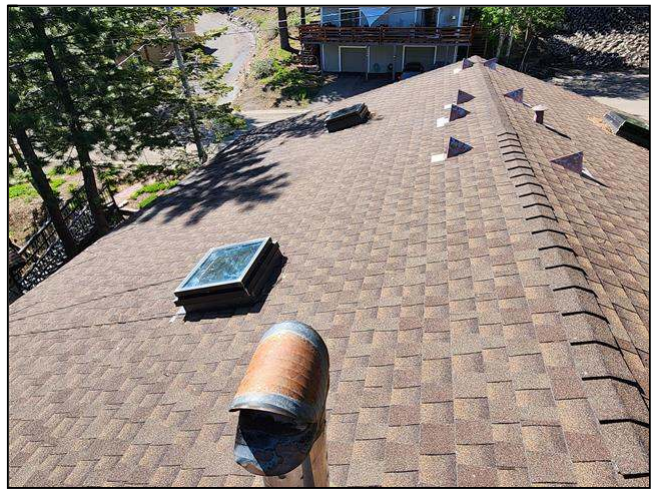
2.0 Item 2(Picture) view of roof
