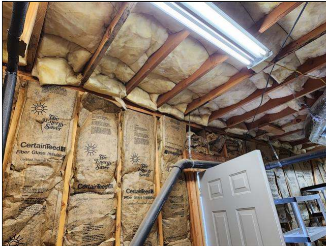
8.1 Item 1(Picture) view of subfloor insulation
