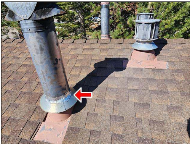
2.3 Item 1(Picture) flue pipes sealed well
