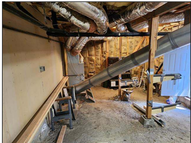
3.0 Item 2(Picture) view of crawlspace
