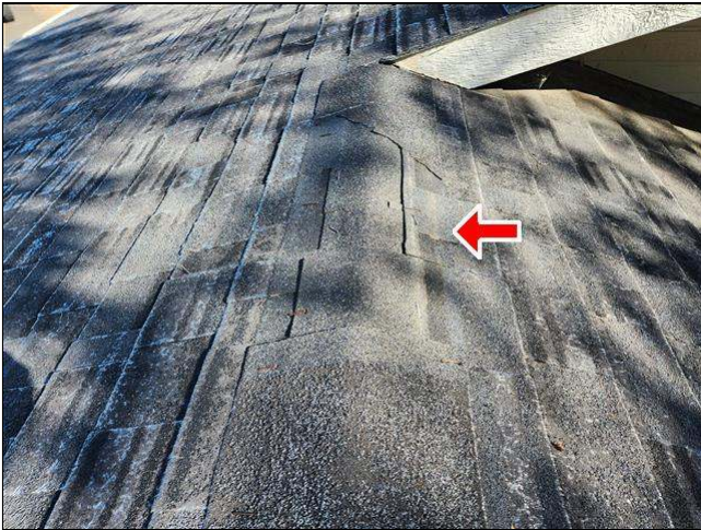
2.1 Item 5(Picture) missing ridge cap shingles
