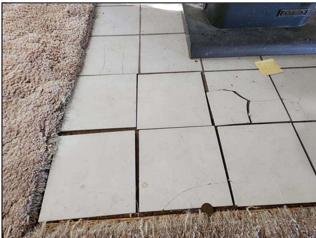
11.3 Item 3(Picture) cracked/loose tiles
