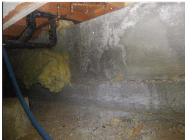
9.1 Item 2(Picture) falling foundation insulation
