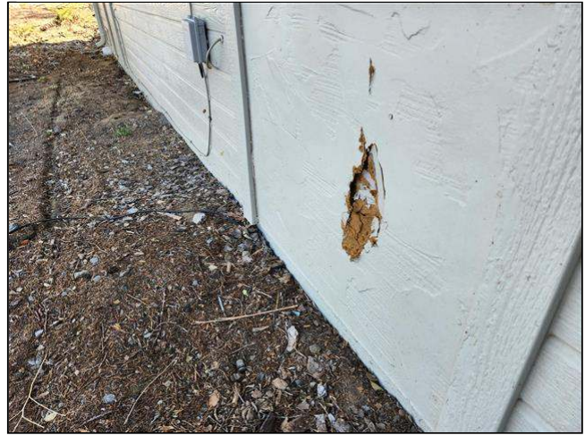
7.2 Item 2(Picture) impact damage at west wall
