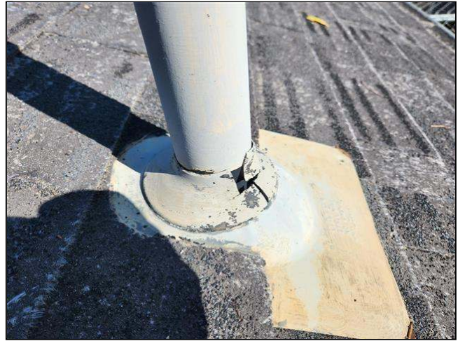
2.3 Item 2(Picture) failing boot seals
