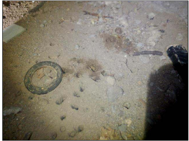
5.7 Item 2(Picture) moisture drips from subfloor under shower
