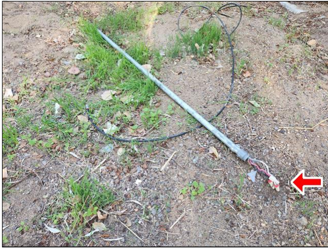
4.5 Item 1(Picture) loose wire ends at south exterior
