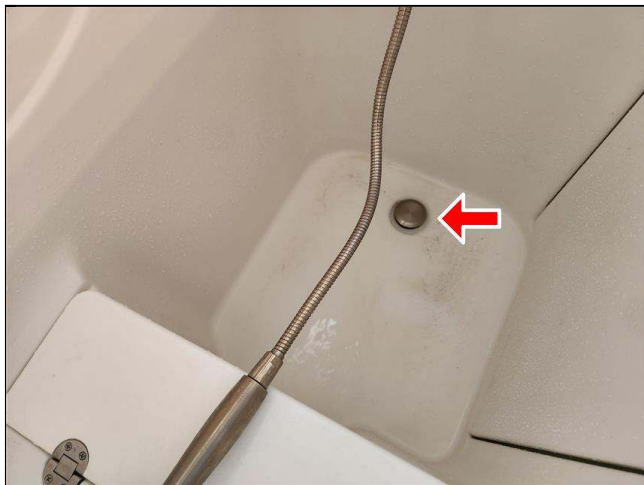
5.5 Item 1(Picture) drain plug does not hold
