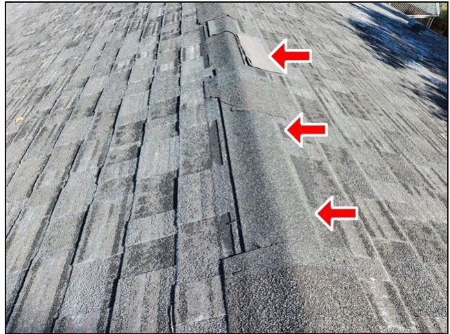
2.1 Item 6(Picture) missing ridge cap shingles
