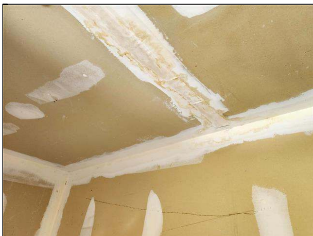
1.9 Item 3(Picture) signs of moisture intrusion
