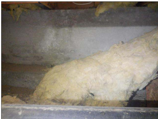
9.1 Item 1(Picture) falling foundation insulation
