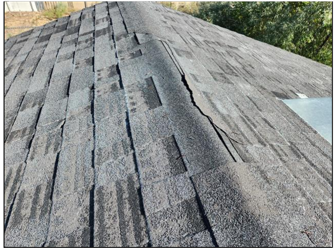
2.1 Item 8(Picture) missing ridge cap shingles
