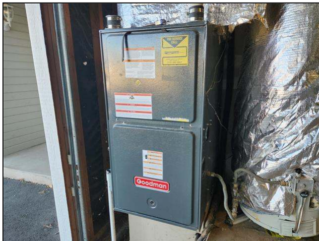
10.0 Item 1(Picture) forced air furnace
