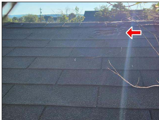
1.9 Item 6(Picture) damaged roofing shingles
