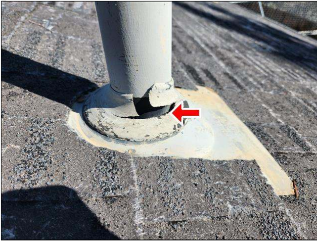
2.3 Item 1(Picture) failing boot seals
