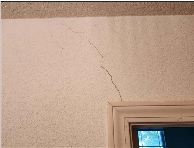
7.2 Item 3(Picture) settlement crack at hallway
