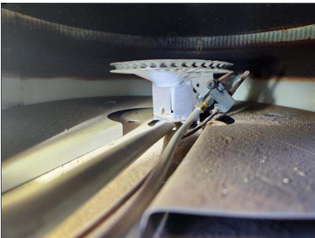
5.4 Item 3(Picture) water heater burner compartment
