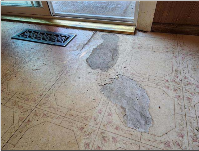
7.3 Item 5(Picture) worn/damaged flooring
