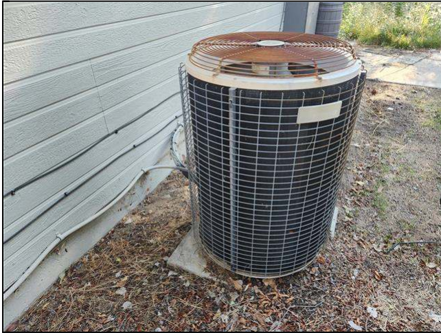
10.4 Item 1(Picture) condensing unit
