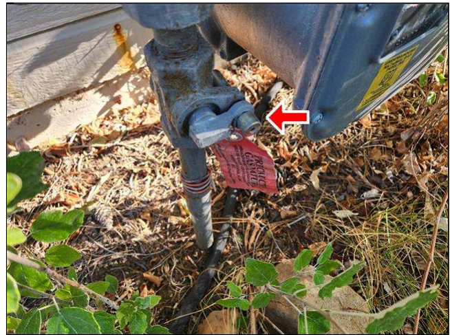
5.11 Item 2(Picture) main fuel shut-off valve
