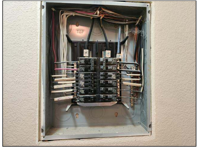
4.1 Item 4(Picture) laundry room panel conductors
