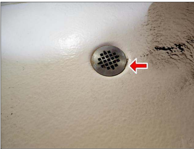
5.7 Item 3(Picture) possibly leaking around shower drain
