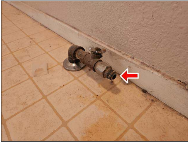
5.10 Item 1(Picture) dryer gas valve uncapped
