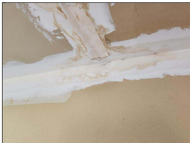
1.9 Item 4(Picture) signs of moisture intrusion
