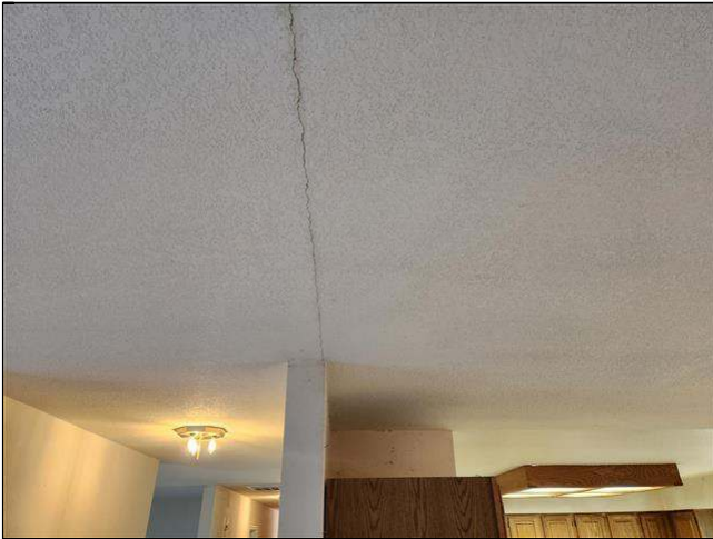
7.1 Item 2(Picture) hairline settlement cracks at ceilings
