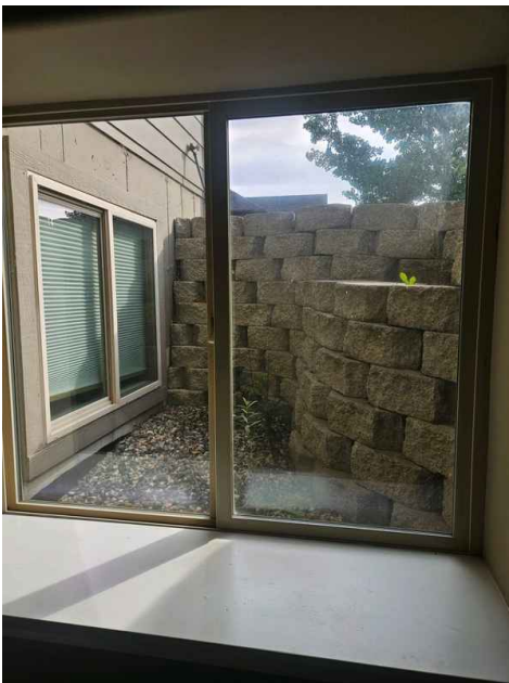
Basement Living Room South
