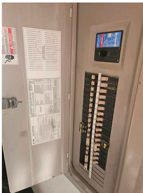
Main & Subpanels, Service & Grounding, Main Overcurrent Device: Panel Manufacturer Cutler Hammer
