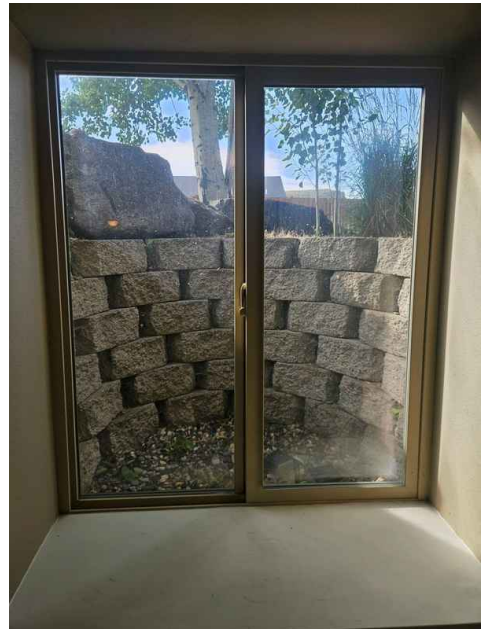
Basement Living Room South
