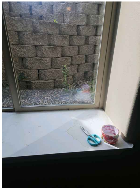
Basement Living Room South
