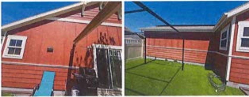
Walkways, Patios & Driveways: Driveway, Patio, Walkway Material Concrete
