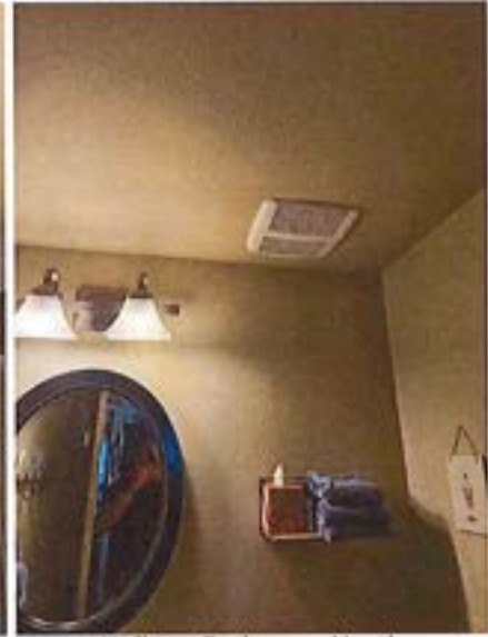
Hallway Bathroom North
