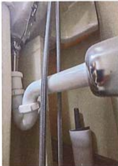
North Hallway Bathroom
