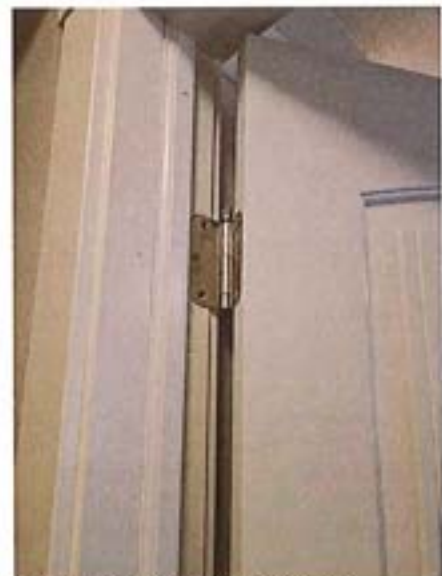
Basement Southeast Bedroom
