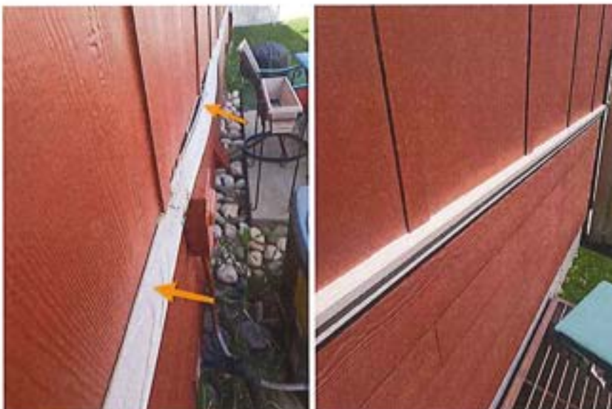
Z Flashing At Transition North
