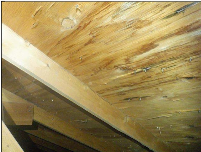
3.9 Item 1(Picture) moisture stains from past leaks
