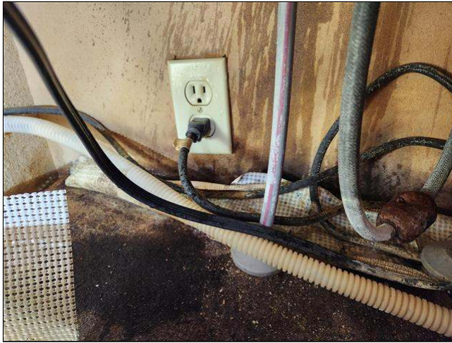
5.4 Item 3(Picture) leaking under kitchen sink
