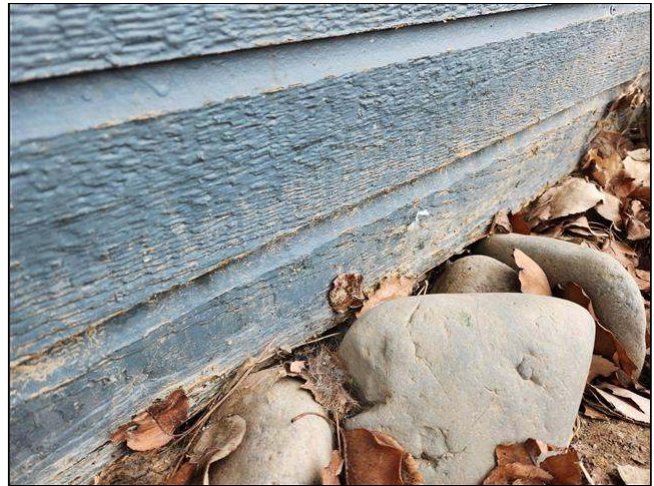
1.1 Item 4(Picture) damaged lower edge at north side
