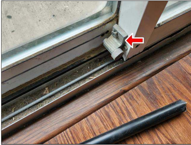
1.3 Item 1(Picture) broken lock at master sliding glass door
