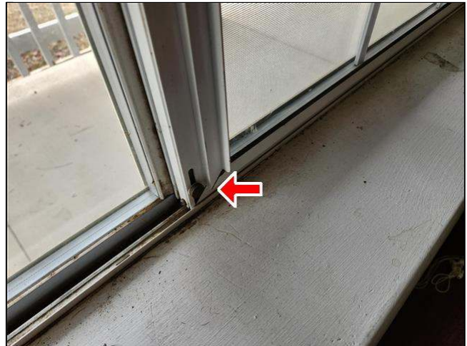
1.4 Item 2(Picture) windows secure with secondary lock
