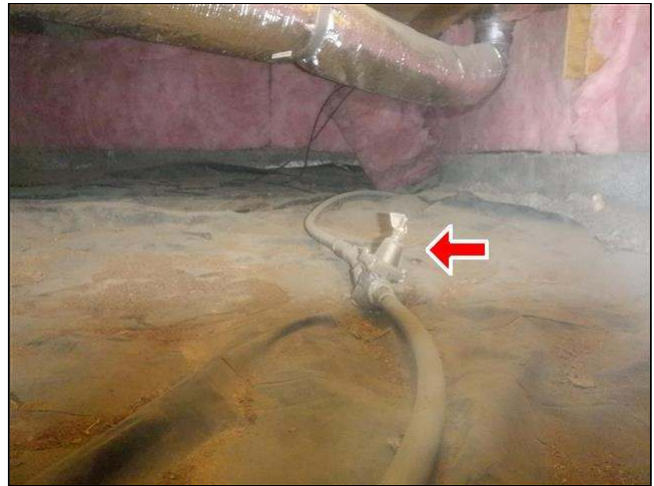
5.1 Item 3(Picture) pressure regulator in crawlspace
