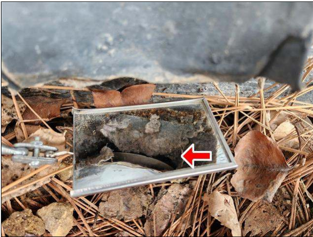
9.4 Item 2(Picture) clogged dryer vent hood
