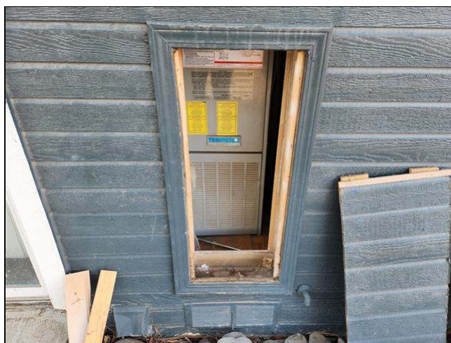
10.0 Item 1(Picture) forced air furnace
