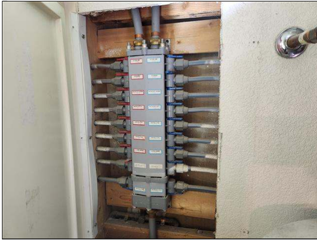
5.1 Item 1(Picture) distribution manifold
