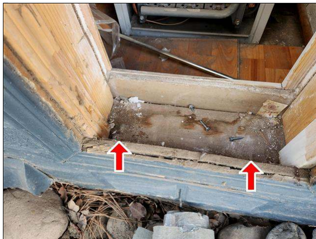
10.0 Item 4(Picture) signs of moisture intrusion inside wall framing
