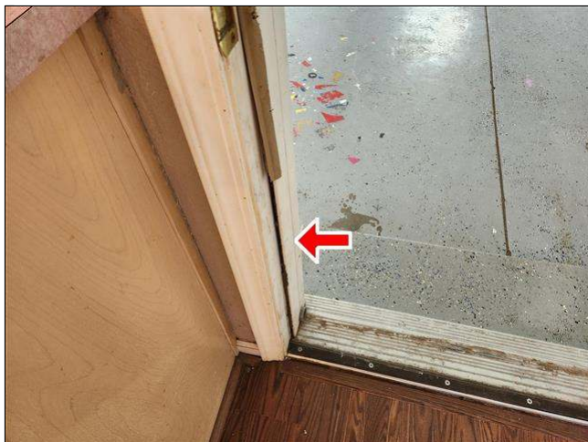
8.8 Item 1(Picture) damaged weather seal at occupant door
