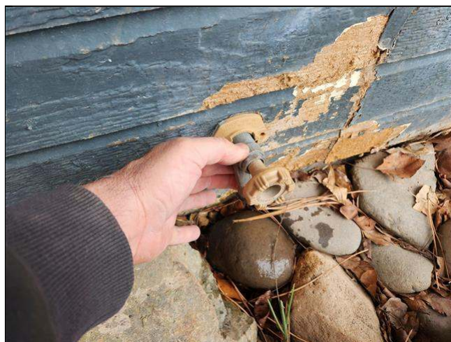
5.0 Item 1(Picture) north hose bib not secured
