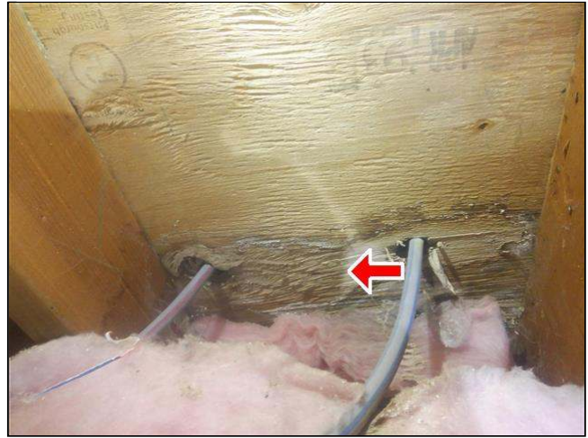
5.4 Item 4(Picture) subfloor under kitchen sink remains solid
