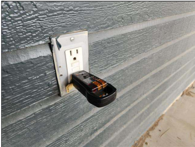
4.7 Item 1(Picture) faulty GFCI at front exterior wall
