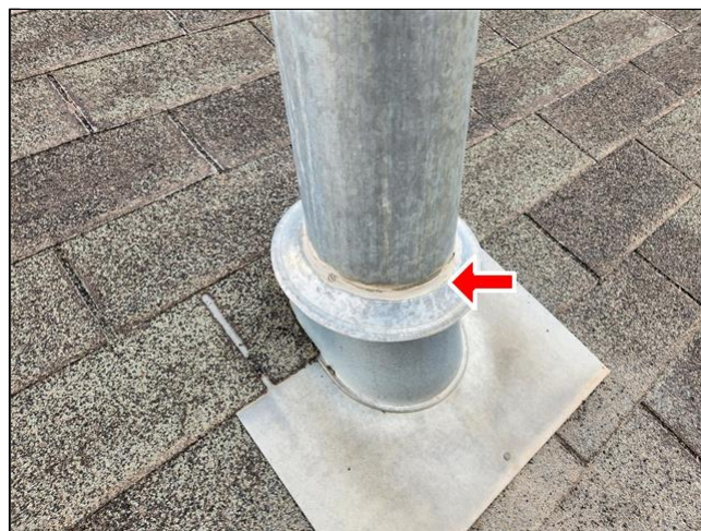
2.3 Item 2(Picture) flue pipes sealed well
