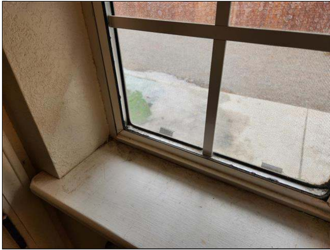
1.4 Item 3(Picture) missing/broken window pane at master bathroom
