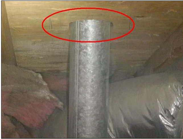
5.7 Item 1(Picture) minimum 1" clearance from combustibles
