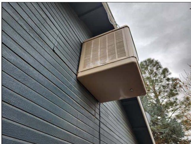
10.4 Item 1(Picture) evaporative cooler
