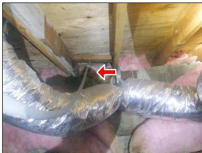
5.0 Item 2(Picture) north hose bib leaks into crawlspace
