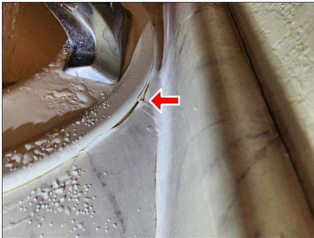
7.3 Item 1(Picture) recommend seal around master bath sink
