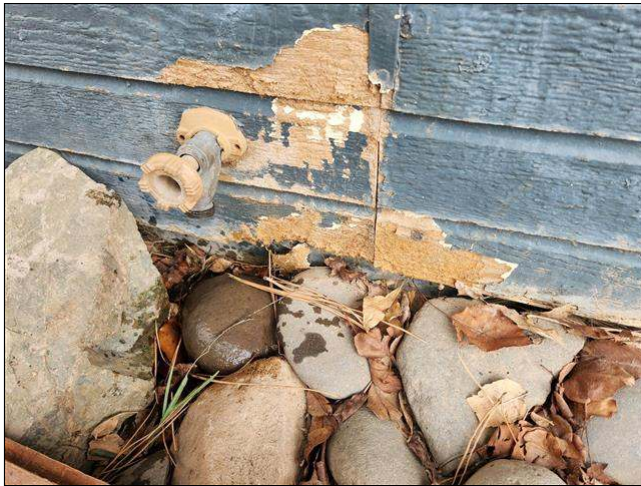
1.1 Item 3(Picture) damaged wall siding at north side
