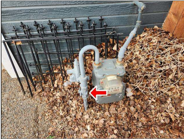
5.10 Item 1(Picture) main fuel shut-off valve
