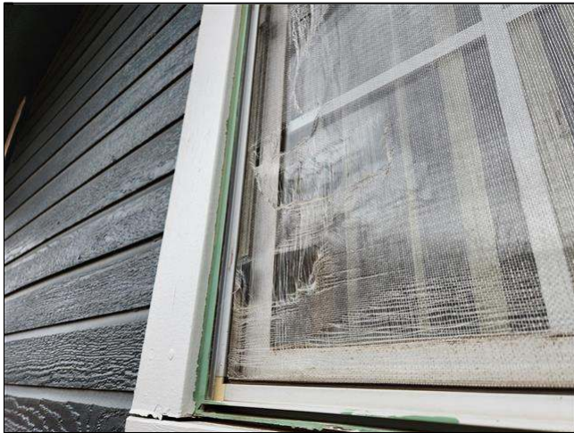
1.4 Item 4(Picture) damaged window screens
