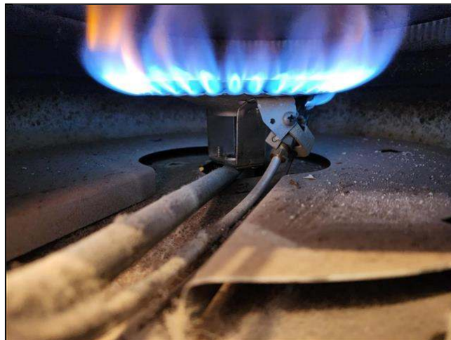
5.3 Item 2(Picture) water heater burner compartment
