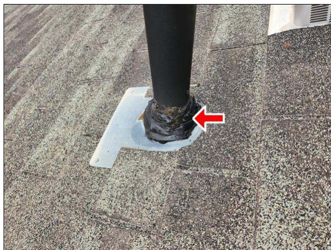
2.3 Item 1(Picture) plumbing vent pipes sealed well
