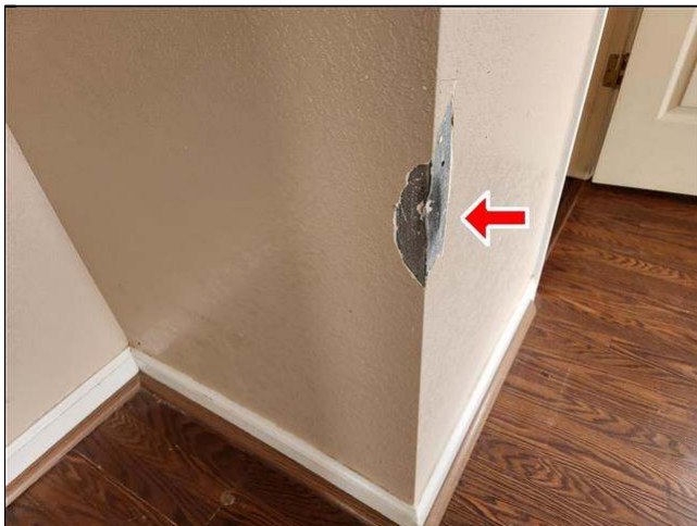
7.1 Item 1(Picture) master bedroom drywall damage
