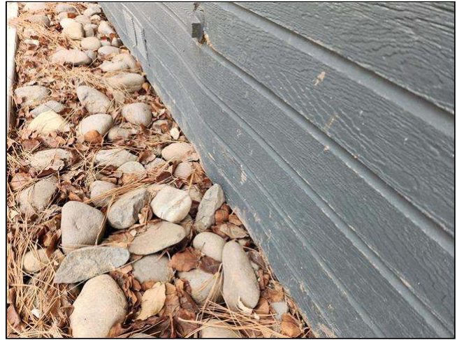
1.1 Item 2(Picture) bowed siding at north side
