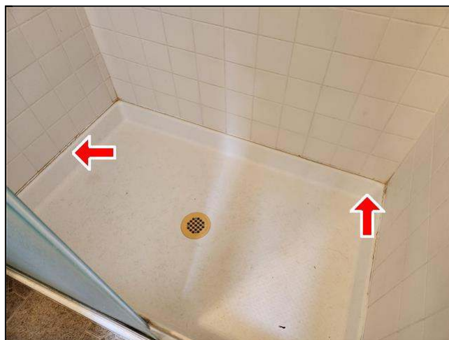
5.6 Item 2(Picture) seal shower enclosures as needed
