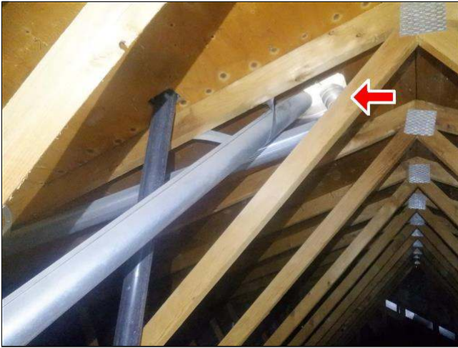
9.4 Item 1(Picture) properly vented to exterior
