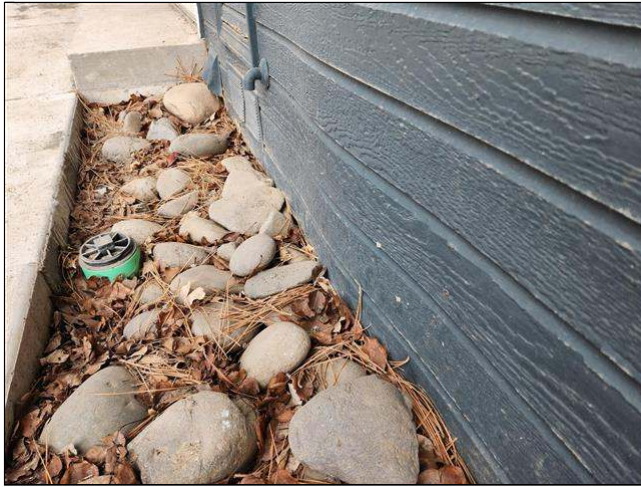
1.1 Item 1(Picture) bowed siding at north side
