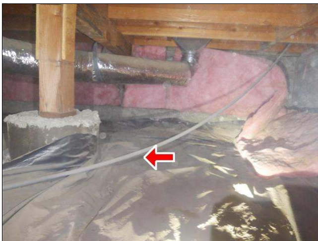
5.1 Item 4(Picture) water supply pipe needs securing
