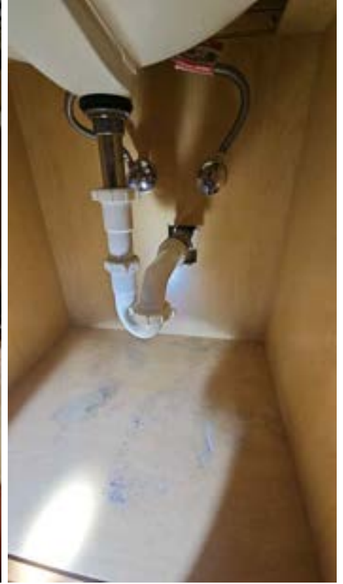
Hallway Bathroom Left
