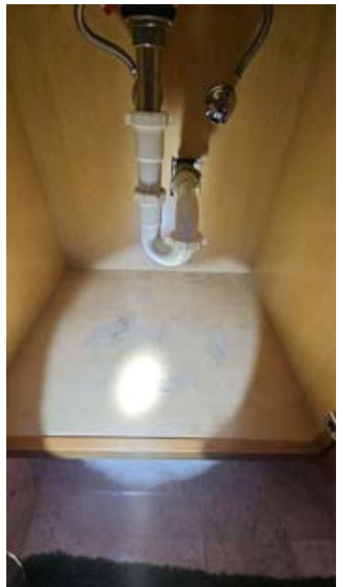
Hallway Bathroom Left
