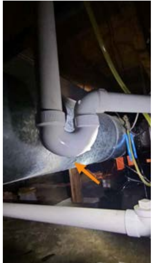
Master Bathroom Crawlspace
