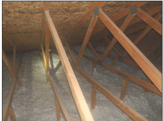
9.0 Item 2(Picture) view of attic insulation
