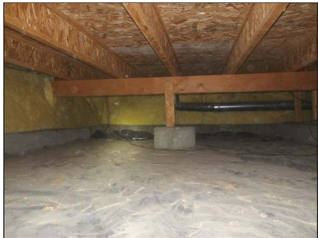
3.0 Item 2(Picture) view of crawlspace
