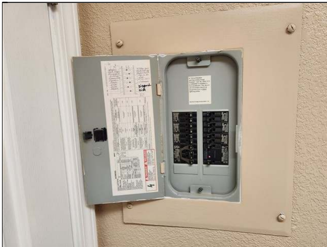
4.1 Item 1(Picture) laundry room panel
