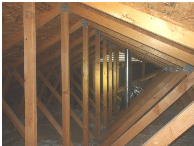
8.11 Item 2(Picture) view of garage roof structure
