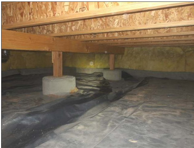
3.0 Item 1(Picture) view of crawlspace
