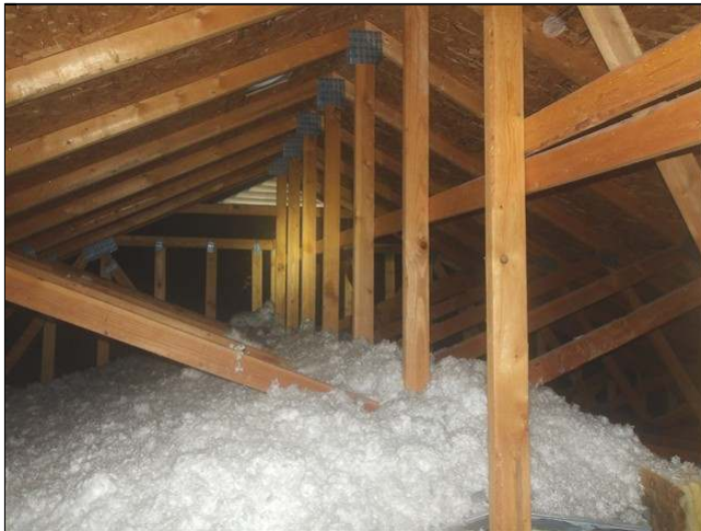
9.0 Item 1(Picture) view of attic insulation
