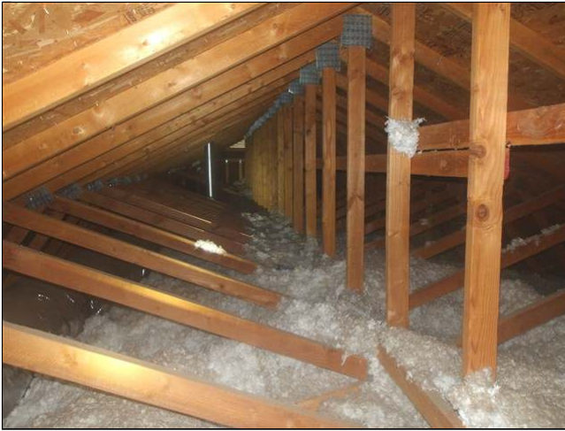
3.8 Item 3(Picture) view of attic
