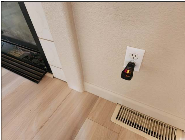
4.6 Item 1(Picture) Hot/Neutral wires are crossed (reverse polarity)
