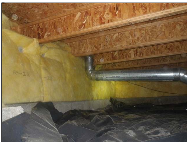
9.1 Item 1(Picture) view of crawlspace insulation
