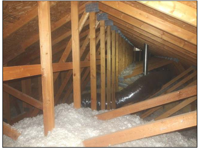
3.8 Item 4(Picture) view of attic
