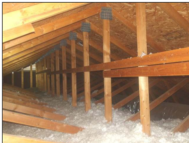
3.8 Item 2(Picture) view of attic
