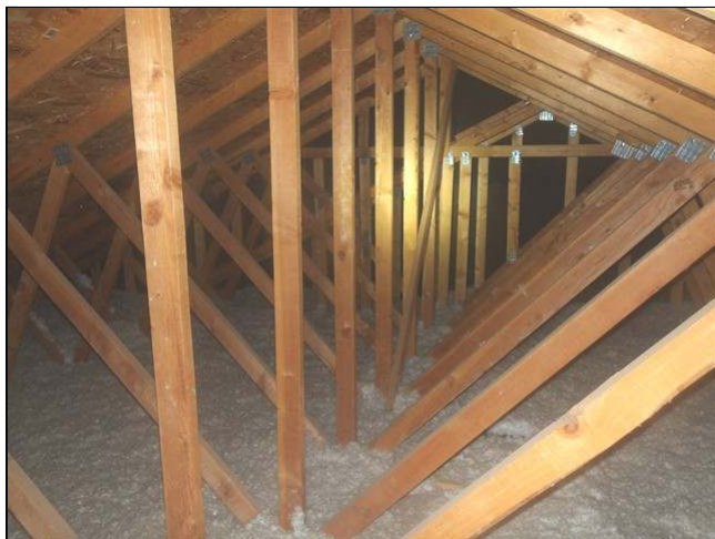
8.11 Item 1(Picture) view of garage roof structure
