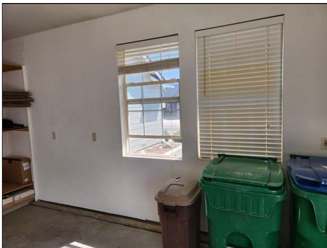
1.4 Item 1(Picture) North window at garage East wall
