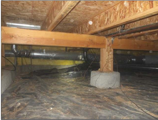
3.0 Item 3(Picture) view of crawlspace
