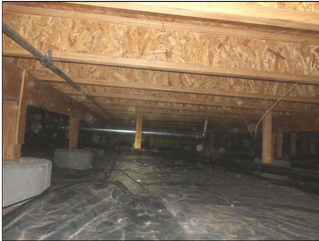
3.0 Item 5(Picture) view of crawlspace
