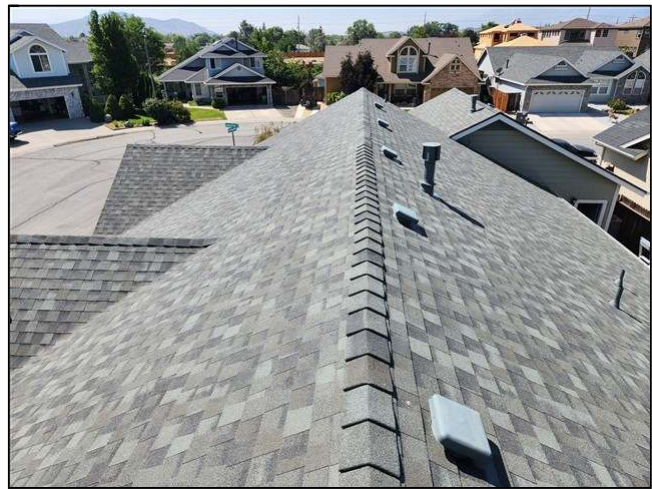
2.0 Item 2(Picture) view of roof
