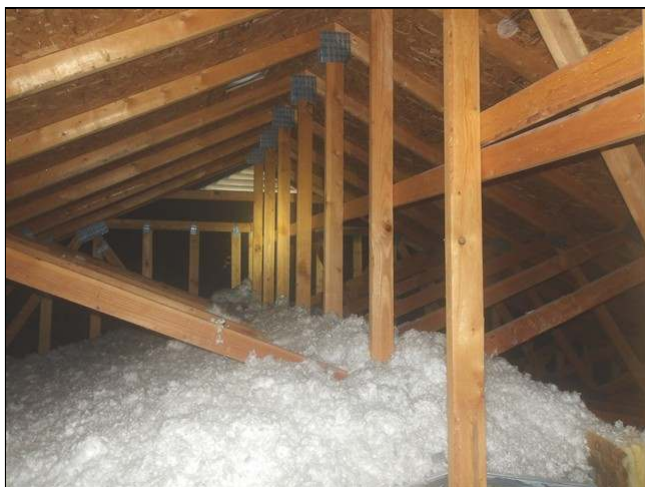
3.8 Item 1(Picture) view of attic
