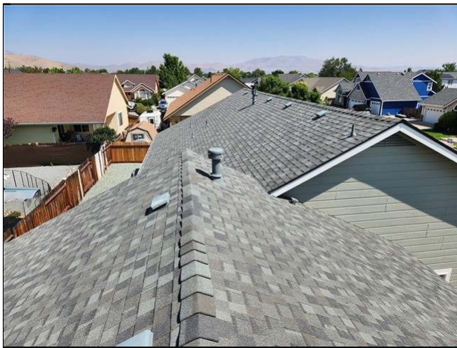
2.0 Item 1(Picture) view of roof
