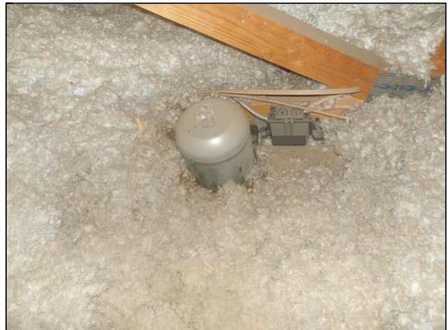
9.0 Item 4(Picture) contacting insulation
