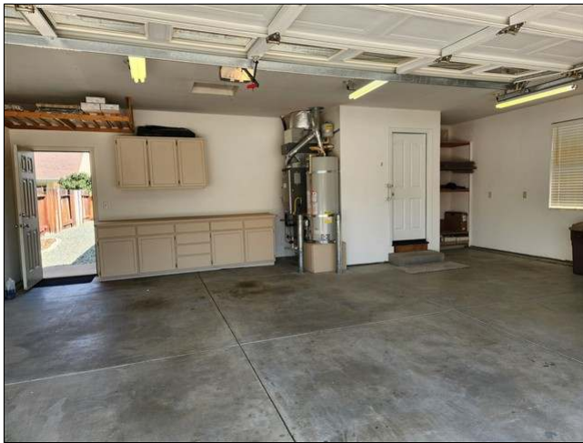
8.0 Item 1(Picture) view of garage
