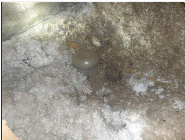
9.0 Item 5(Picture) contacting insulation
