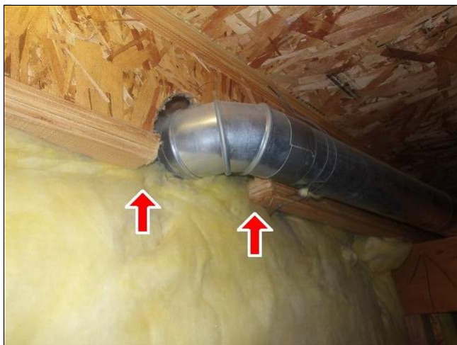
3.6 Item 1(Picture) bottom cord has been cut through
