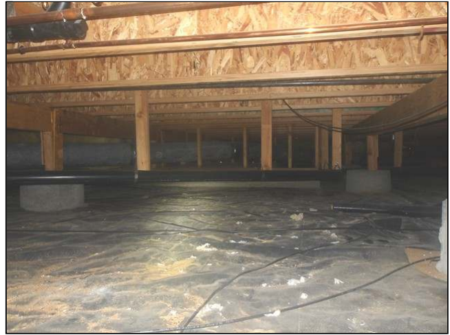
3.0 Item 4(Picture) view of crawlspace
