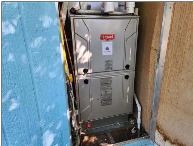
9.0 Item 1(Picture) forced air furnace
