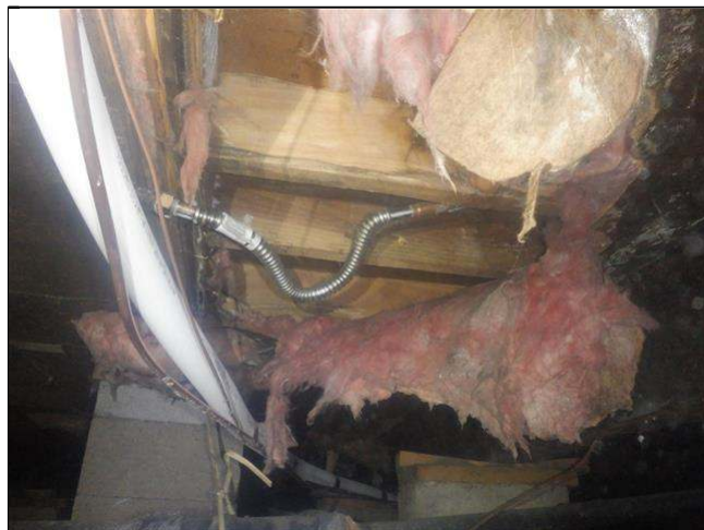
8.1 Item 1(Picture) floor insulation under laundry area
