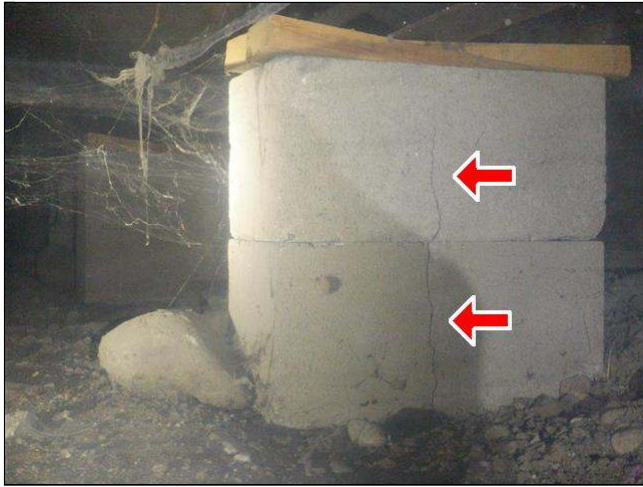
3.4 Item 3(Picture) cracked blocks under laundry area
