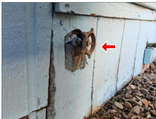
5.0 Item 1(Picture) main water shut-off valve
