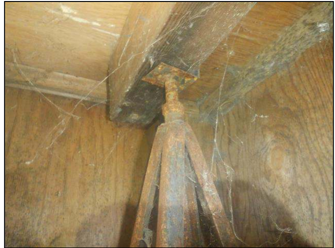
8.3 Item 4(Picture) rusted metal screw jack
