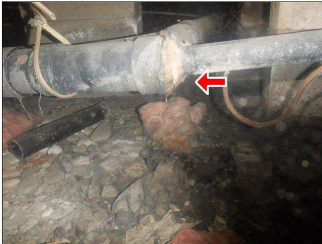
5.3 Item 1(Picture) leaking plumbing drain pipe
