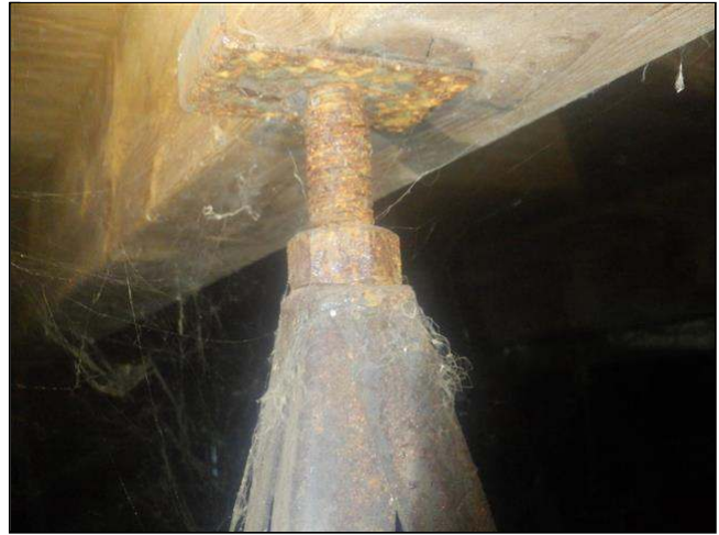
8.3 Item 2(Picture) rusted screw jacks
