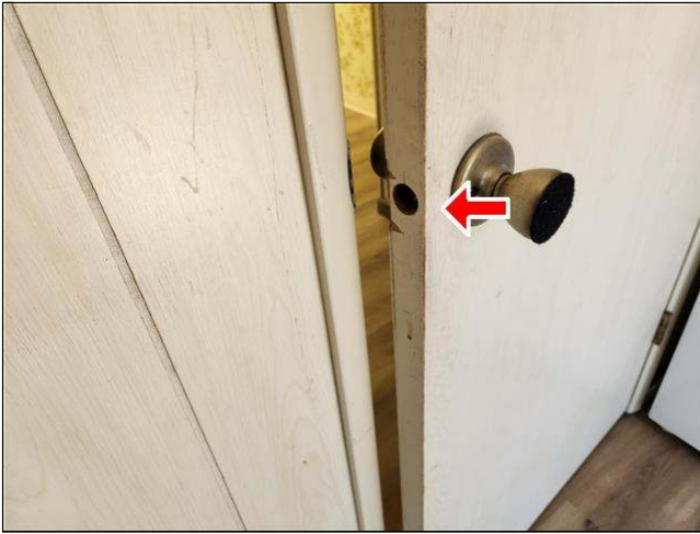
7.5 Item 1(Picture) door missing striker
