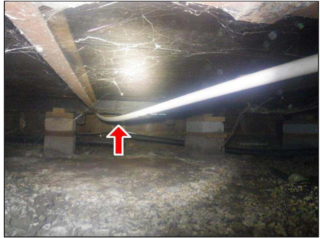
9.0 Item 4(Picture) unsupported, sagging condensate drain line
