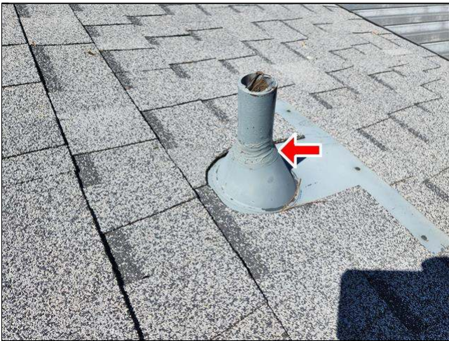
2.3 Item 1(Picture) plumbing vent pipes sealed well
