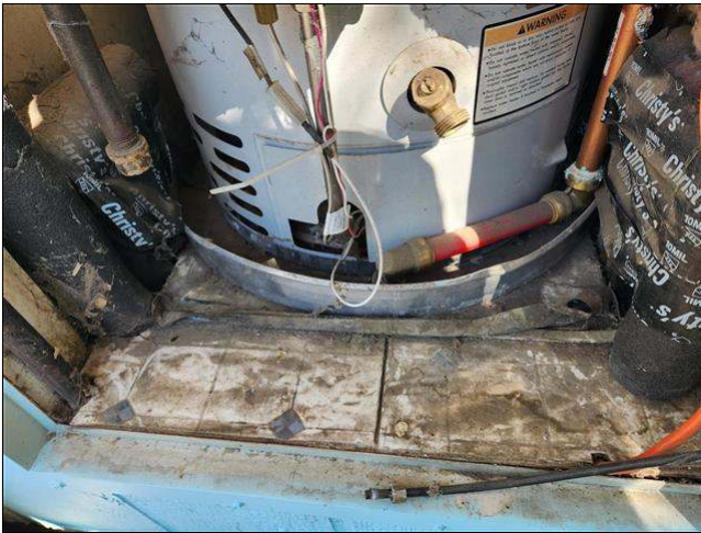
5.4 Item 3(Picture) setting in a drip pan
