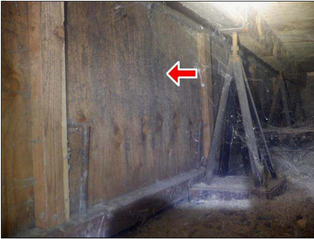
8.3 Item 1(Picture) signs of poor ventilation
