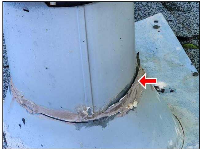
2.3 Item 2(Picture) recommend seal flue pipe flashing
