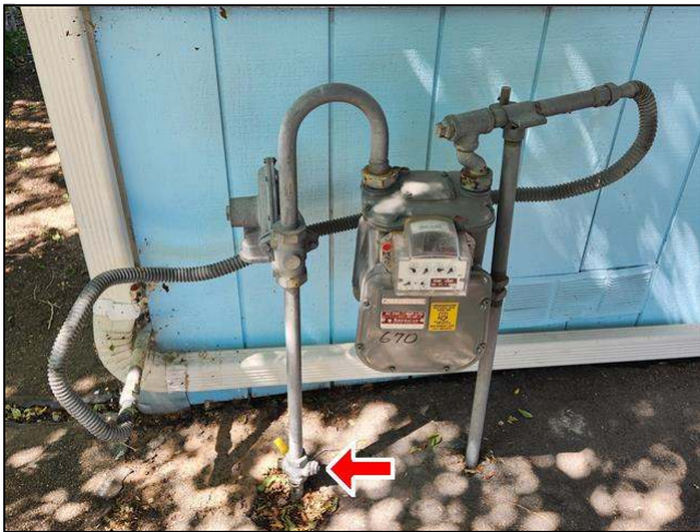
5.11 Item 1(Picture) main fuel shut-off valve
