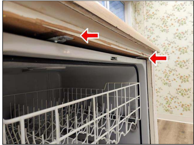
6.1 Item 2(Picture) upper mounts missing fasteners
