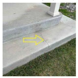
2.5.3 Backfill soil under concrete patio to prevent damage, promote stability, and deter pest entry. **(Exterior South)**
