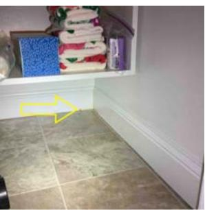
11.2.3 Further investigate cause and extent of staining/damage and correct as required. No moisture detected at time of inspection. (Basement Living Room)
