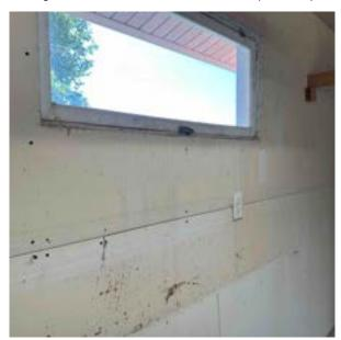
6.6.3 Further investigate cause and extent of wall staining and repair as required to prevent further damages. No moisture detected at time of inspection. **(Shop)**
