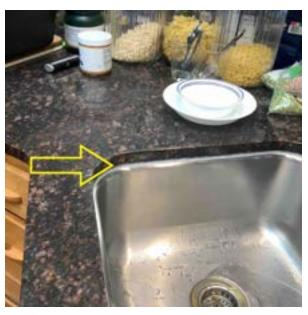
11.7.5 Secure countertop to cabinets to promote stability and prevent further damages. (2nd Floor Hallway Bathroom)
