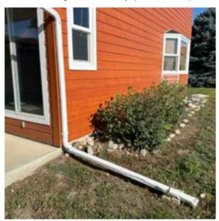
2.1.4 Provide clearance from landscaping to siding/wood contact to prevent deterioration and deter pest entry. **(Exterior East)**
