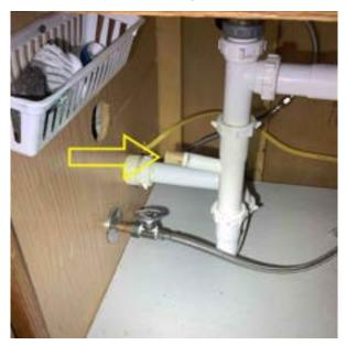
10.3.4 Repair drain line showing signs of leaking to prevent secondary water damages.
