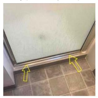
10.9.5 Seal all cracks/gaps/joints in and around tubs and showers to reduce water penetration and subsequent deterioration. (1st Floor Hall Bathroom)
