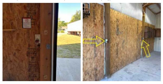
8.8.4 Replace missing switch plate/junction box cover to prevent electrical hazards. (Garage)
