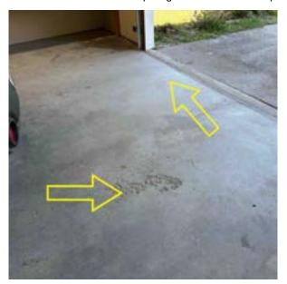
6.5.2 Consult qualified contractor to evaluate settled/improperly sloped/cracked concrete floor and repair as required to promote intended drainage and prevent secondary water damages. (**Shop**)
