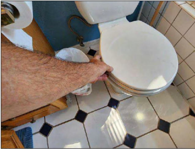
5.4 Item 2(Picture) master bathroom toilet
