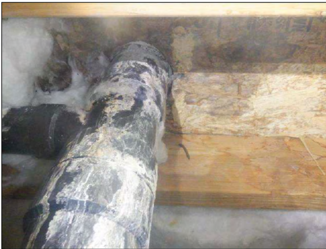
5.4 Item 4(Picture) subfloor remains solid
