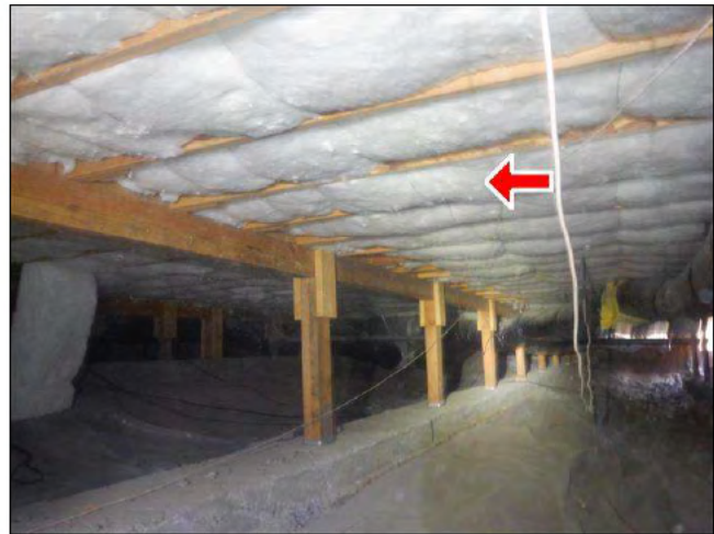
9.0 Item 2(Picture) view of subfloor insulation
