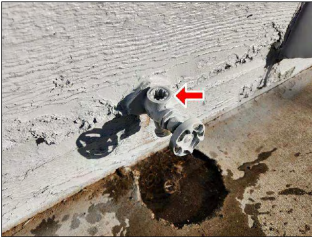
5.0 Item 1(Picture) south exterior hose bib
