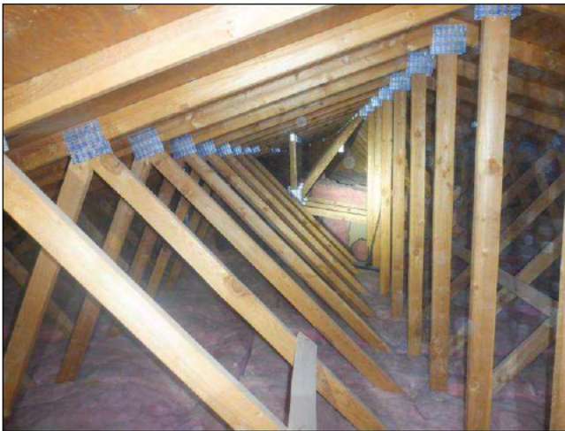
3.8 Item 3(Picture) view of attic
