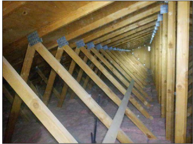
3.8 Item 2(Picture) view of attic
