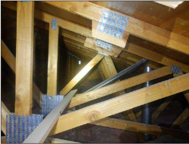
3.8 Item 1(Picture) view of attic
