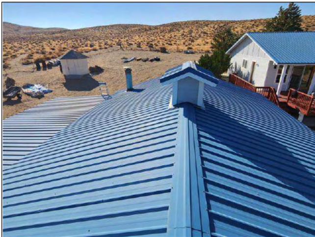
8.10 Item 1(Picture) view of garage roof
