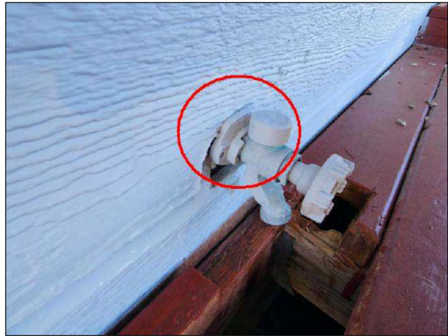
5.0 Item 2(Picture) secure north hose bib flange
