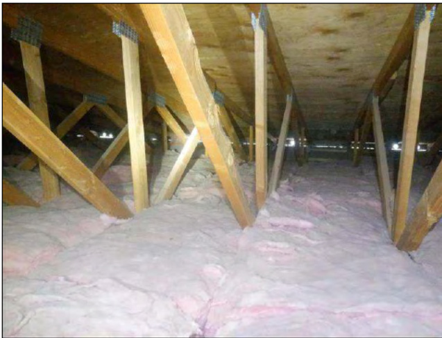
9.0 Item 1(Picture) view of attic insulation
