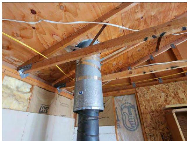
8.14 Item 3(Picture) clearances to combustibles
