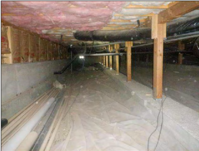
3.0 Item 1(Picture) view of crawlspace
