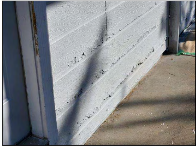
1.1 Item 2(Picture) south side siding boards
