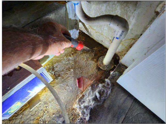
10.0 Item 4(Picture) subfloor remains solid
