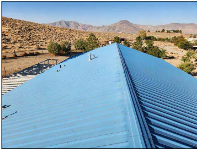
2.0 Item 1(Picture) view of roof
