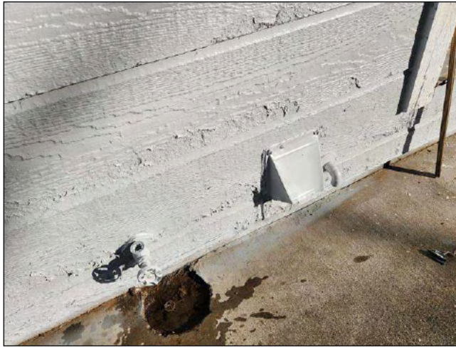
1.1 Item 1(Picture) south side siding boards
