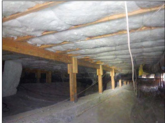
3.0 Item 2(Picture) view of crawlspace
