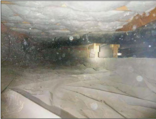
3.0 Item 3(Picture) view of crawlspace
