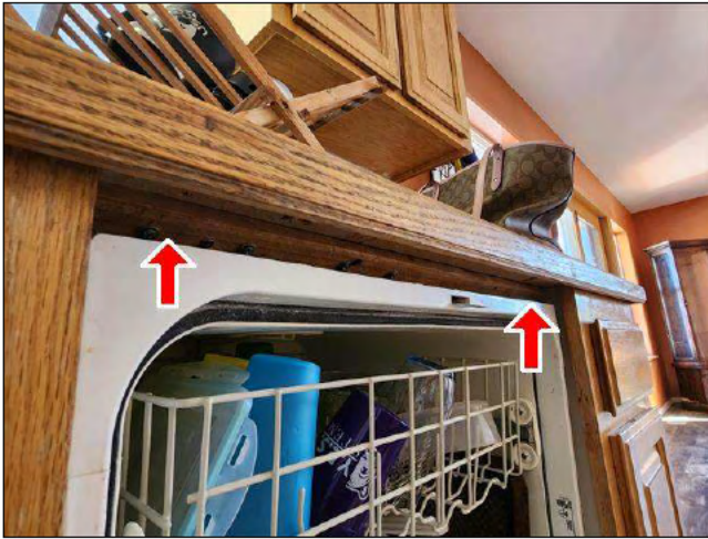
6.1 Item 1(Picture) secure upper dishwasher mounts
