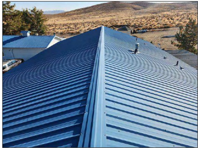
2.0 Item 2(Picture) view of roof
