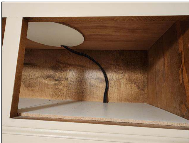
4.5 Item 1(Picture) exposed wire inside cabinet
