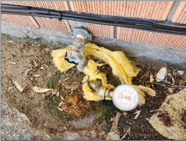
5.2 Item 1(Picture) water pressure at rear hose bib
