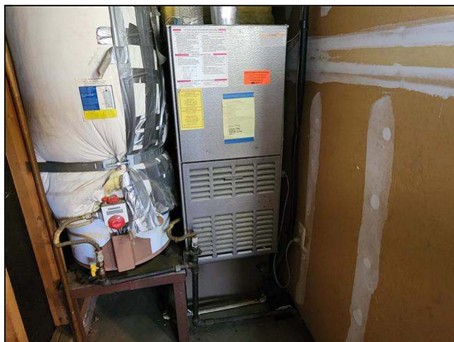
10.0 Item 1(Picture) forced air furnace
