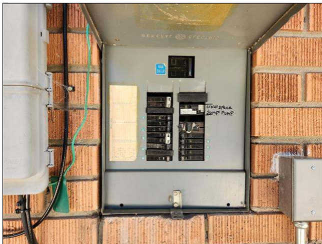
4.1 Item 1(Picture) main electrical panel
