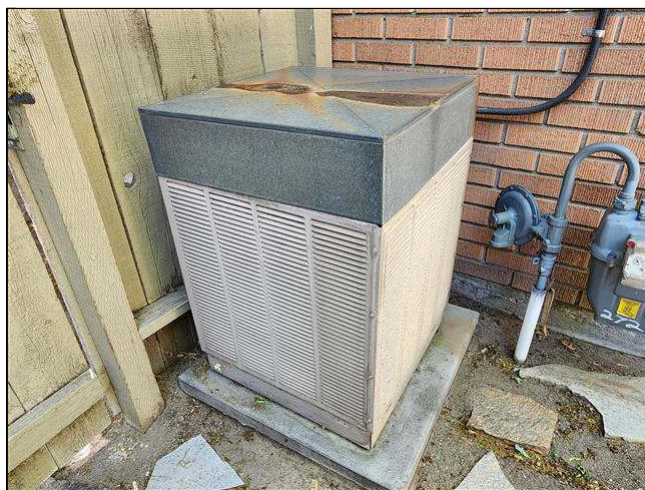
10.5 Item 1(Picture) condensing unit
