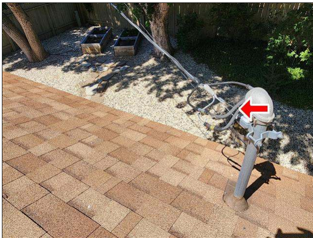
4.0 Item 1(Picture) proper drip loop
