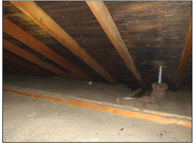
9.3 Item 2(Picture) blackened roof sheathing plywood
