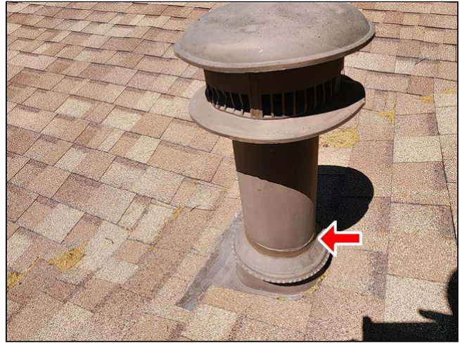
2.3 Item 2(Picture) flue pipes well sealed
