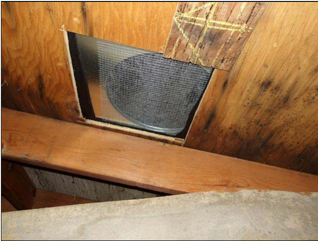
9.3 Item 3(Picture) roof vents recently installed
