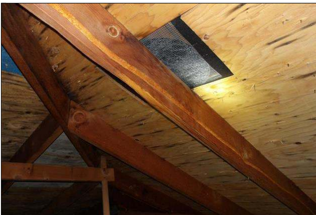
3.9 Item 1(Picture) cracked roof rafter
