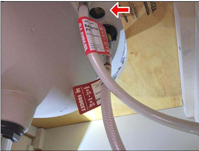
5.5 Item 1(Picture) faucet leaks under base
