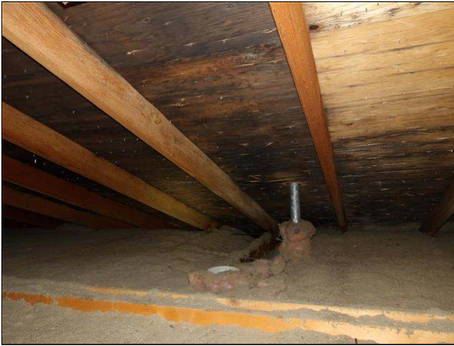
9.3 Item 1(Picture) blackened roof sheathing plywood
