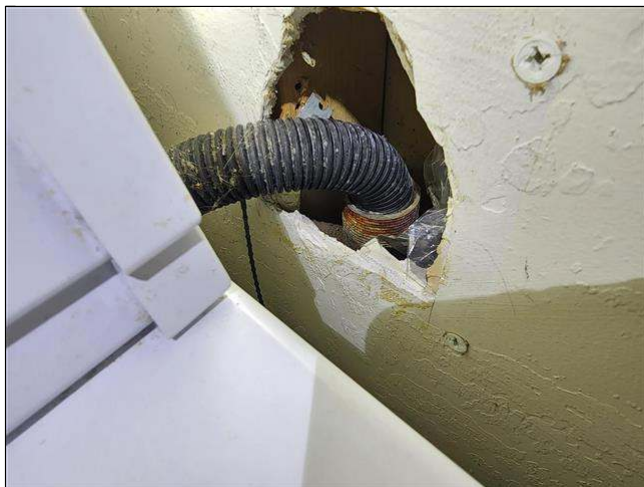
7.2 Item 1(Picture) hole at laundry closet wall
