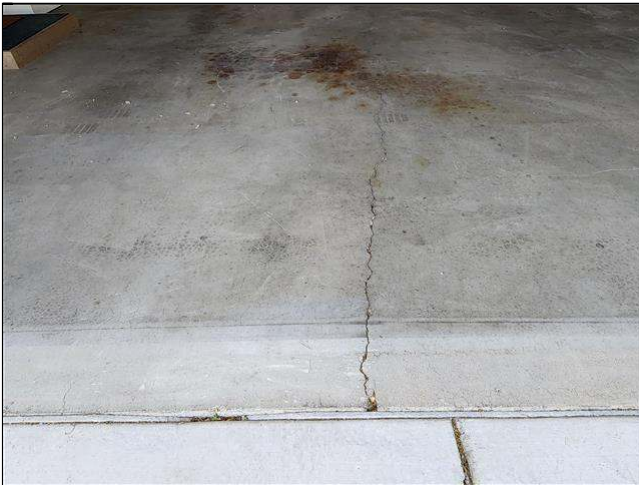
8.4 Item 1(Picture) normal settlement cracks
