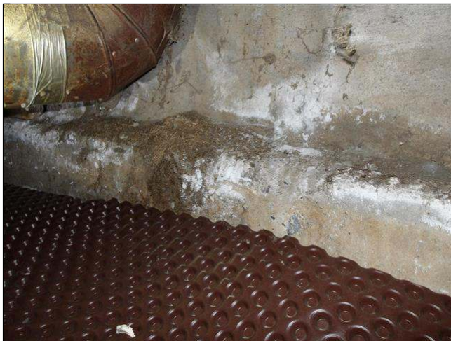
3.2 Item 2(Picture) signs of excessive exterior moisture
