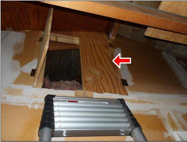
8.3 Item 1(Picture) compromises fire-separation wall integrity
