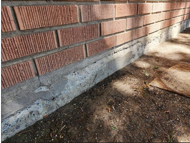
3.2 Item 1(Picture) spalling damage at foundation
