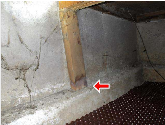
3.4 Item 1(Picture) original support under girder posts
