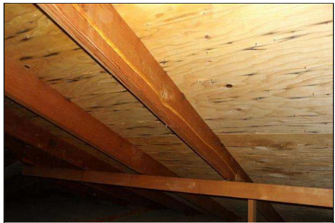
3.9 Item 2(Picture) cracked roof rafter
