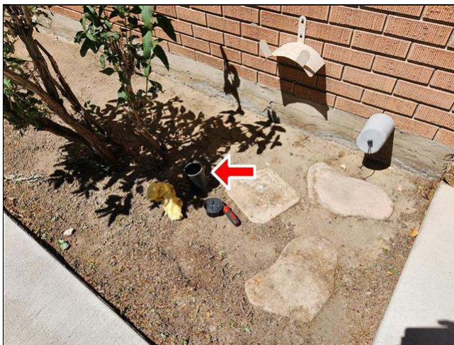
5.0 Item 1(Picture) main water shut-off valve location
