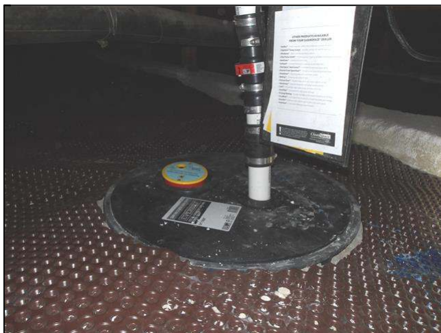
5.12 Item 1(Picture) sump pump in crawlspace area
