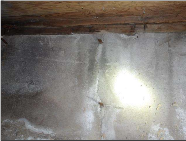
3.2 Item 3(Picture) small vertical foundation crack
