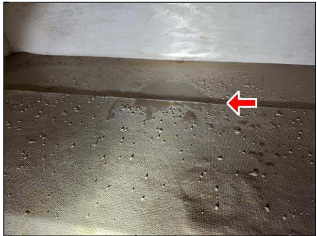
5.5 Item 2(Picture) moisture from leak
