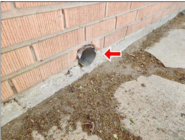
9.4 Item 1(Picture) dryer vent hood missing
