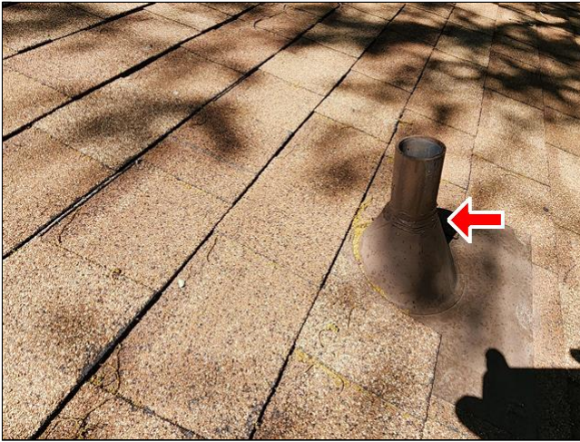
2.3 Item 1(Picture) plumbing vent pipes sealed well
