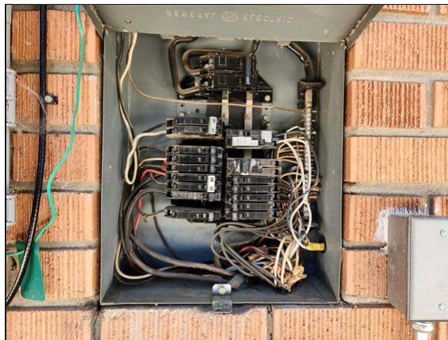
4.1 Item 2(Picture) main panel conductors
