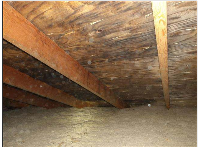
9.3 Item 4(Picture) blackened roof sheathing plywood
