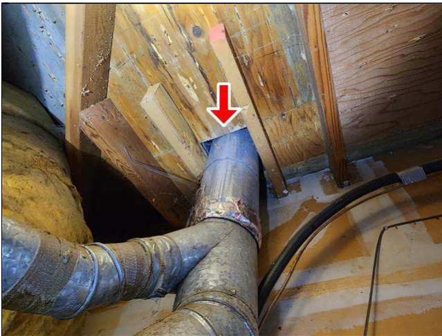
5.8 Item 1(Picture) improper clearance at flue pipe
