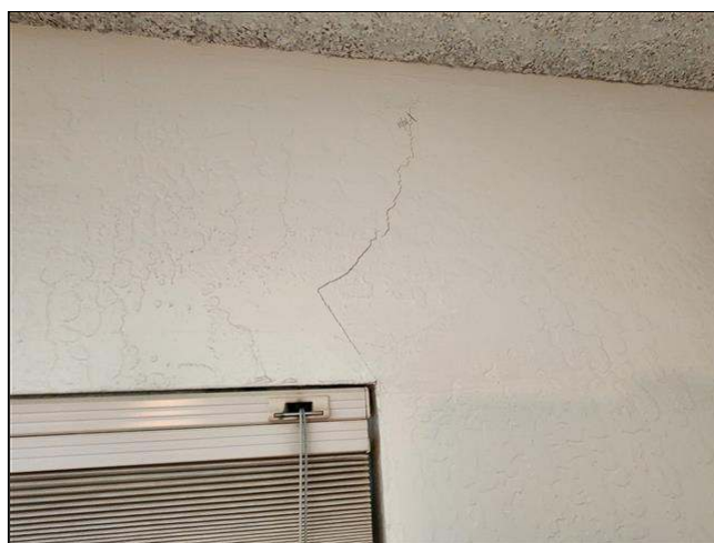
7.2 Item 3(Picture) settlement crack at master bedroom
