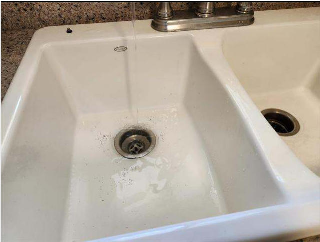
5.3 Item 1(Picture) slow drain at kitchen sink
