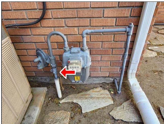
5.11 Item 1(Picture) main fuel shut-off valve
