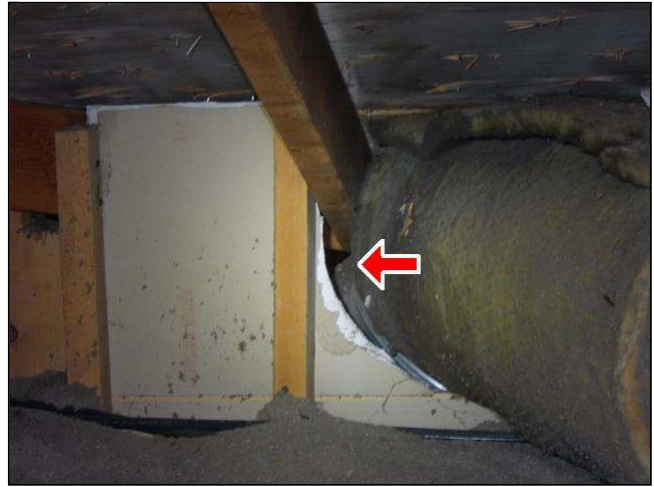
8.3 Item 2(Picture) compromises fire-separation wall integrity
