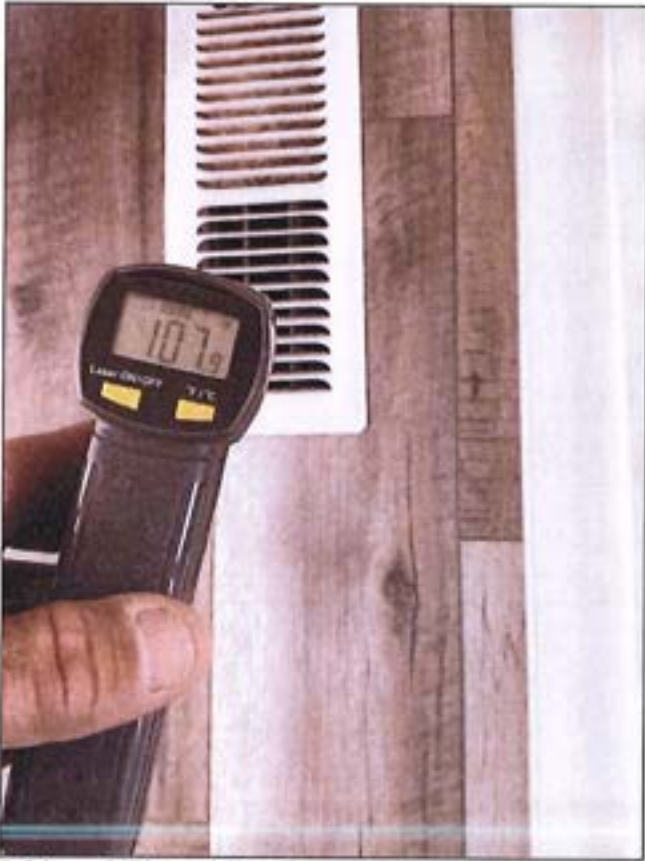
8.0 Item 3(Picture) The furnace temp was 107 F after running 5 minutes.
