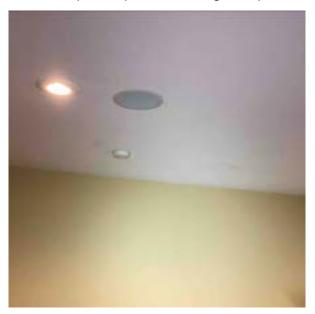
11.2.5 Further investigate cause and extent of staining/damage and correct as required. No moisture detected at time of inspection. (2nd Floor Bathroom)
