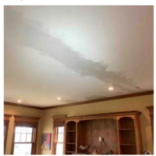
11.2.3 Further investigate cause and extent of staining/damage and correct as required. No moisture detected at time of inspection. (Master Bathroom)
